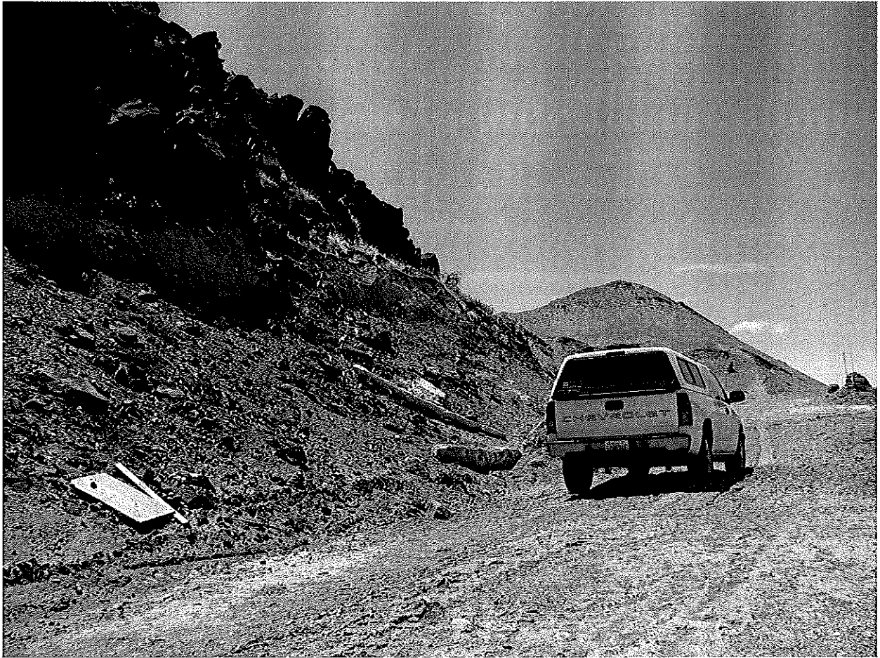
Photo # 3 After – The pickup truck indicates scale after Phase 2 excavation of the basalt outcrop bluff that forms the south wall of bowl in which aluminum waste was disposed.
