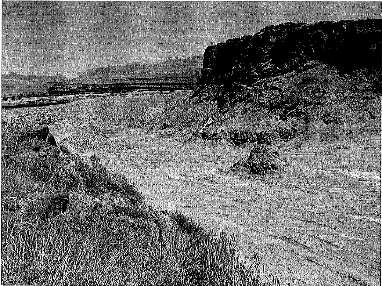
Photo # 1 After Phase 2– The orange pipe in the center indicates the location of the remnant of monitoring well MW-2. The gray aluminum waste below the rock outcropping shows the height of the waste prior to excavation.
