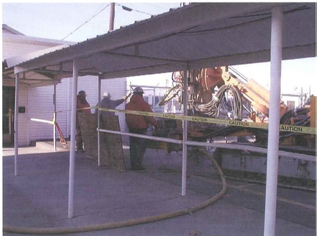
PHOTO 2: LOOKING NORTH WEST AT PREPARATION TO BUILD MONITORING WELL #3
