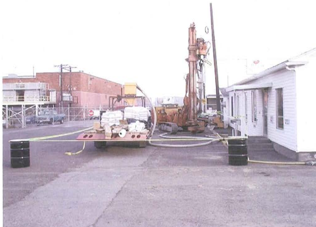
PHOTO 4: LOOKING EAST AT THE CONSTRUCTION OF MONITORING WELL #2
