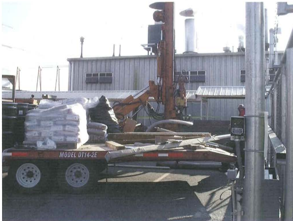
PHOTO 3: DRILLING MONITORING WELL #3, LOOKING EAST
