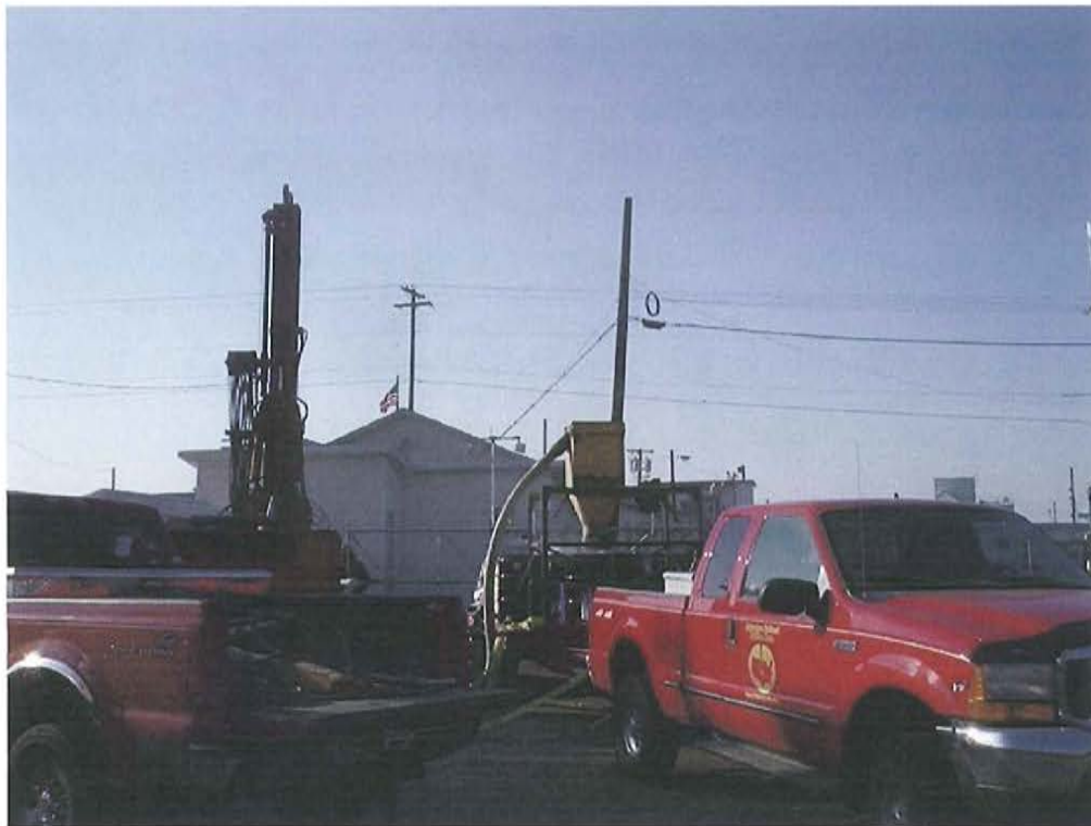
PHOTO 1: LOOKING WEST AT MONITORING WELL #3 CONSTRUCTION
