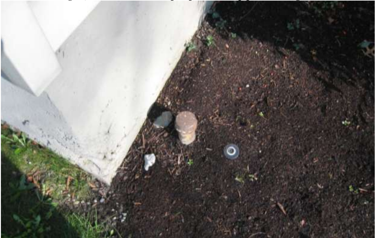
Photo 4: Building 29, Location 7 – close-up of possible fill-pipe remaining
