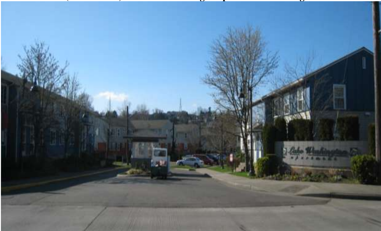
Photo 2: Street (S. Fisher Pl.) at entrance leading to apartments - looking west
