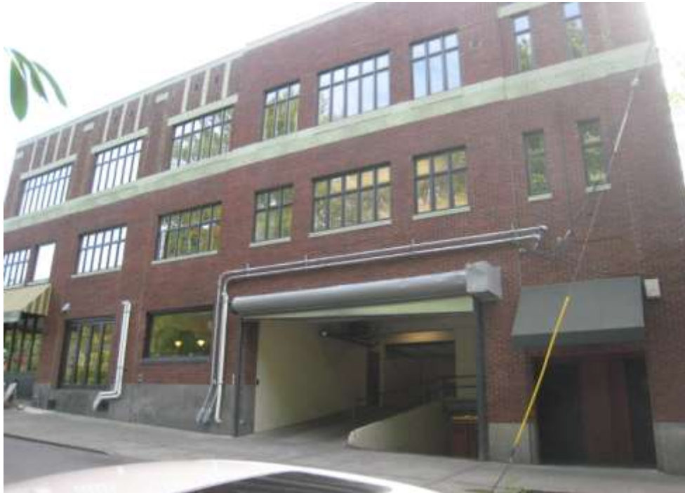
Photo 1: Former Tank Location west side - from the west
