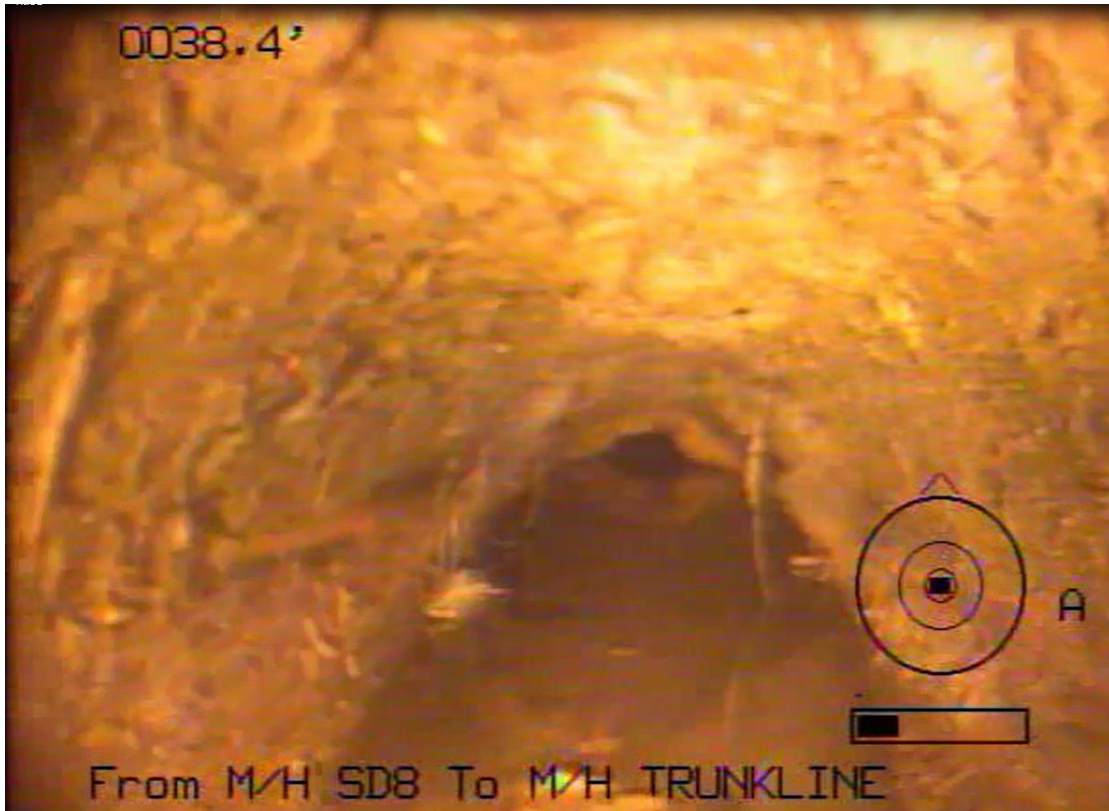
Photo 4: SD-8/SD-9 lateral approaching connection to trunk line.
