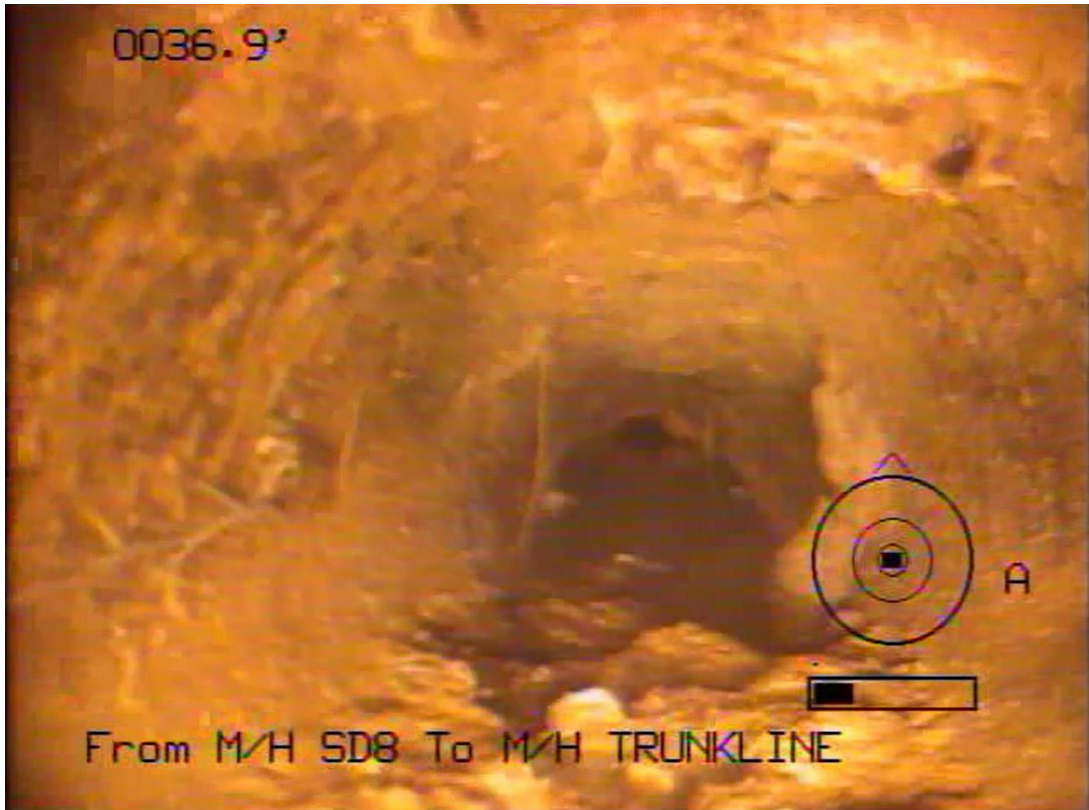
Photo 3. SD-8/SD-9 lateral near connection to trunk line.
