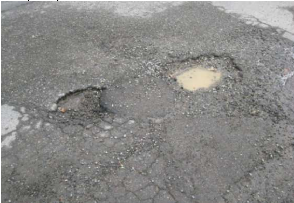
Photo 4: Asphalt in poor condition in front of 4500 4 th S.
