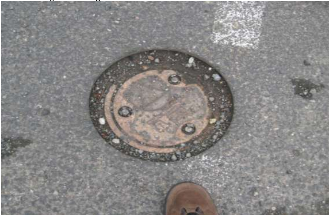
Photo 2: Existing monitoring well in front of 4424 4 th S.
