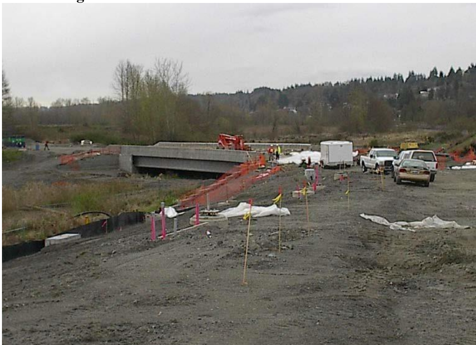
Photo 2: Bridge and Sheet Pile Wall
