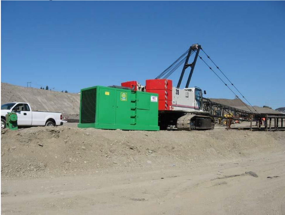
Photo 1: Sheet pile crane
