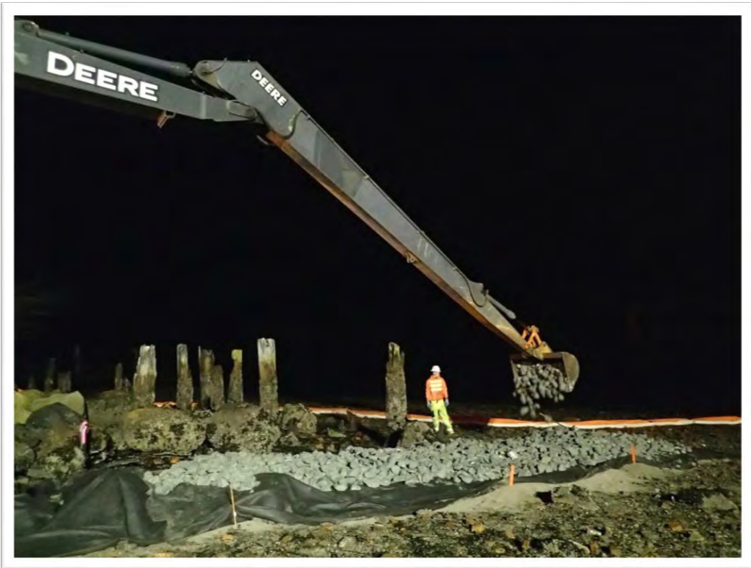
Photo 9: Placement of containment berm
