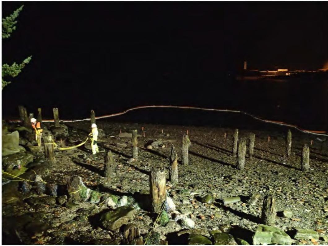
Photo 1: Pre-Construction Condition of the Interim Action Area
