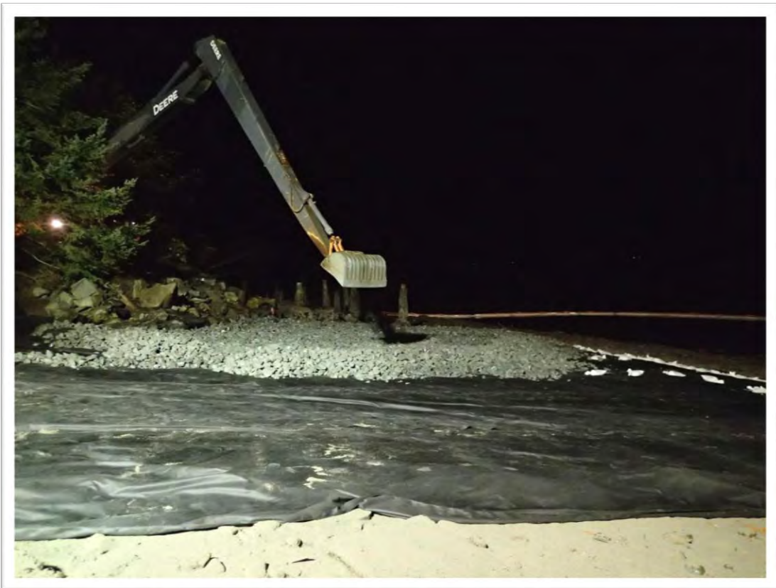
Photo 10: Placement of cap armor
