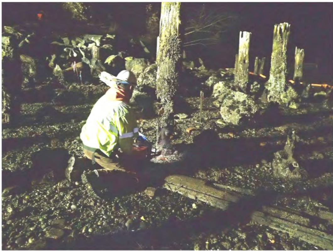
Photo 2: Saw-Cutting of derelict wood piles
