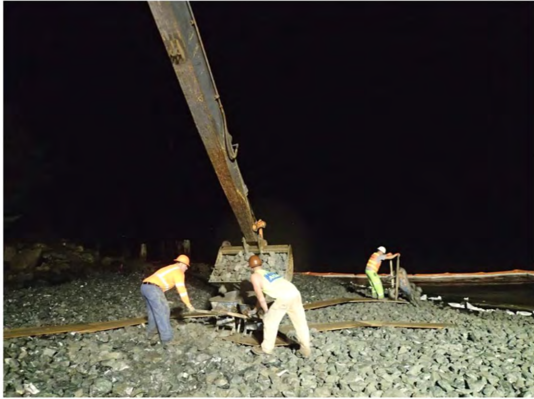
Photo 11: Placement of cap armor
