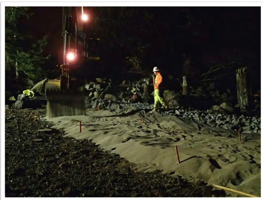
Photo 6: Placement of amended cap (50/50 sand organoclay mix) on prepared mudline
