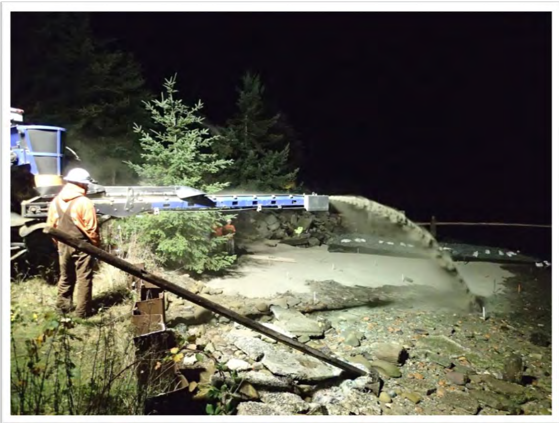
Photo 7: Placement of amended cap (50/50 sand organoclay mix) on prepared mudline
