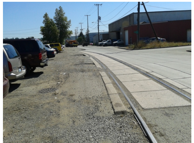
Photograph 6. Easterly view along the South Myrtle Street right-of-way near the former lumber dip tank area.
