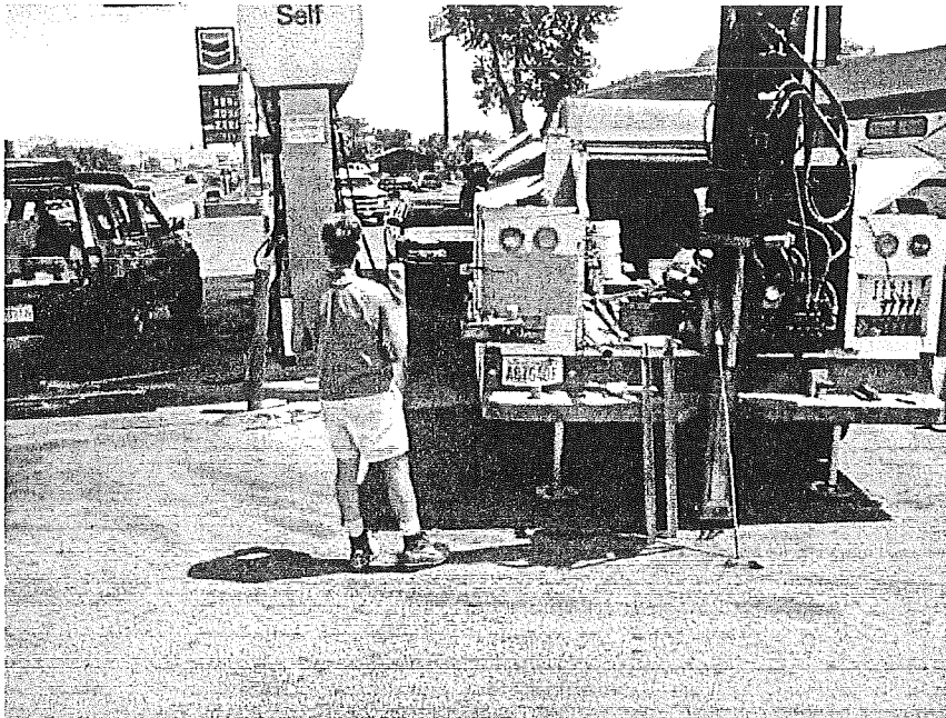
3. Drilling at B2.
