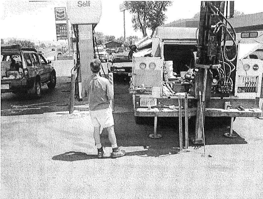
3. Drilling at B2.
