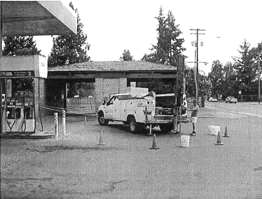
4. Drilling at B4.
