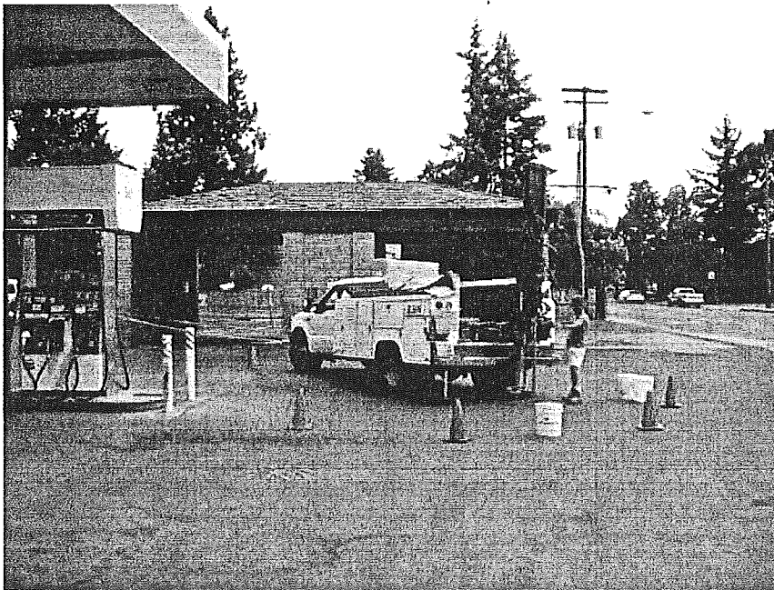
4. Drilling at B4.
