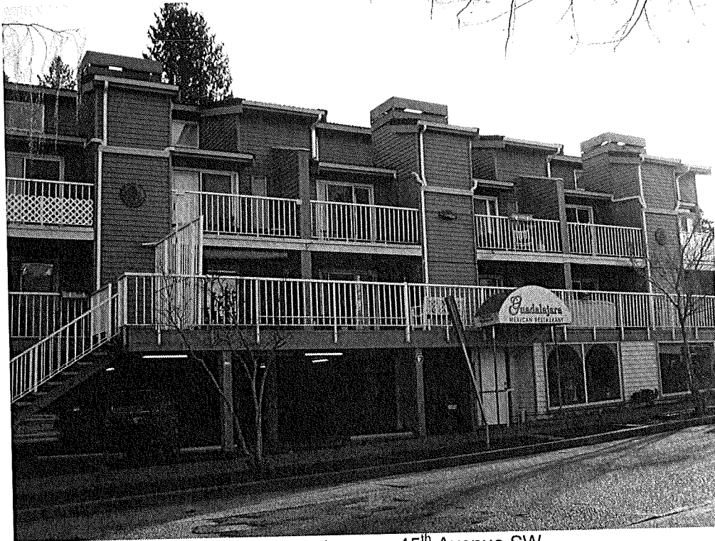
Photo 1 Site building, viewed facing east across 45 th Avenue SW
