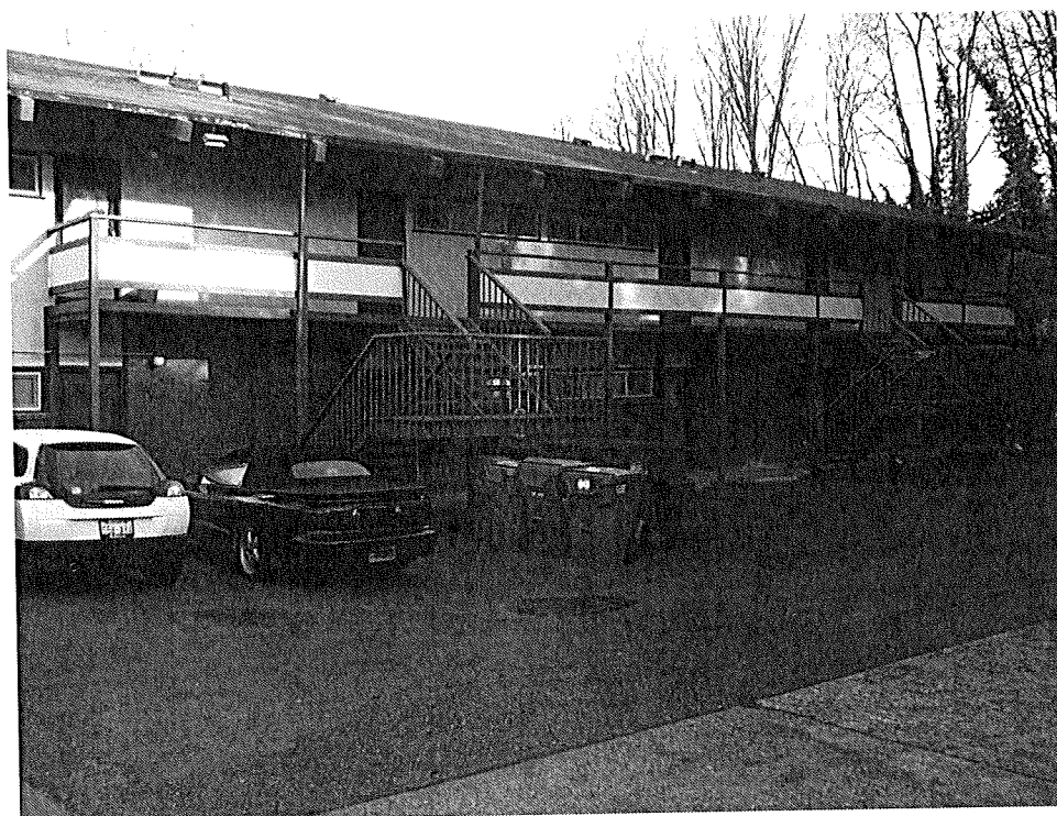
Photo 10 North-adjointing apartment building, viewed facing northeast
