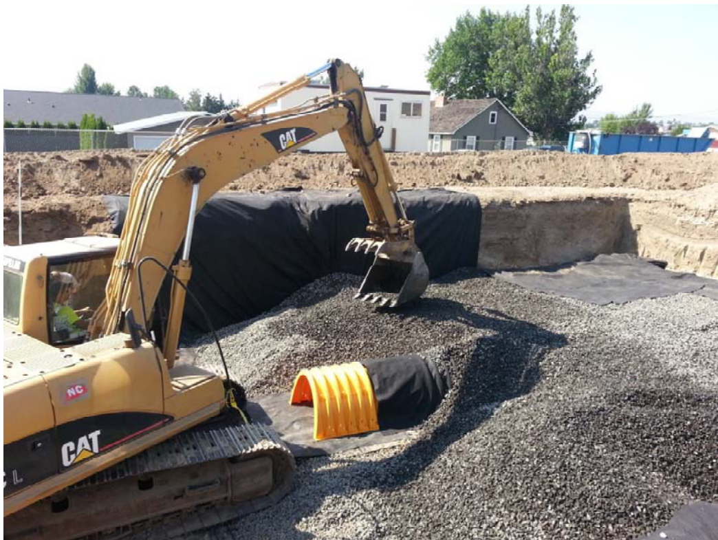
Photo D-8: Apple Valley Elementary School Stormwater Infiltration Gallery under construction.
