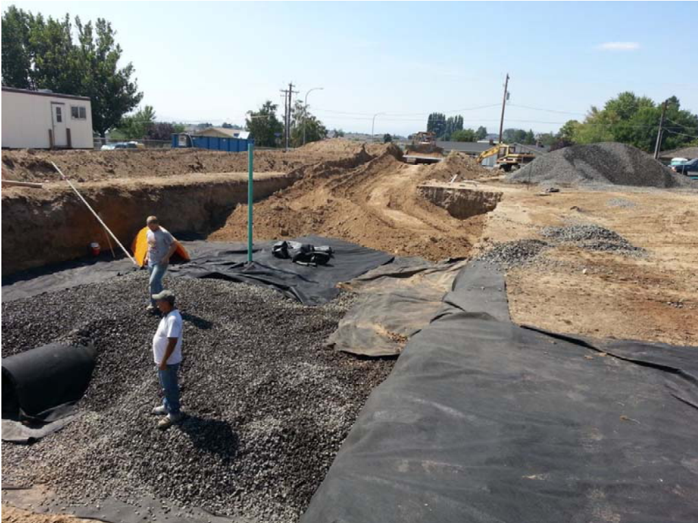
Photo D-7: Apple Valley Elementary School Stormwater Infiltration Gallery under construction.
