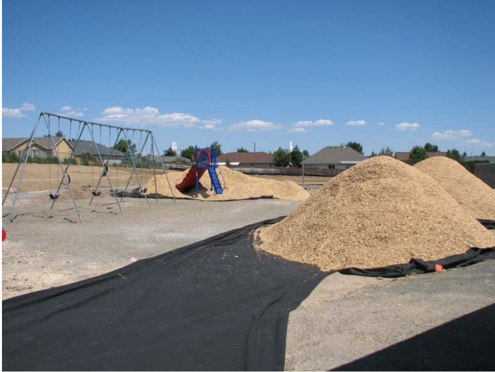
Photo D-5: Apple Valley Elementary School playground area construction.
