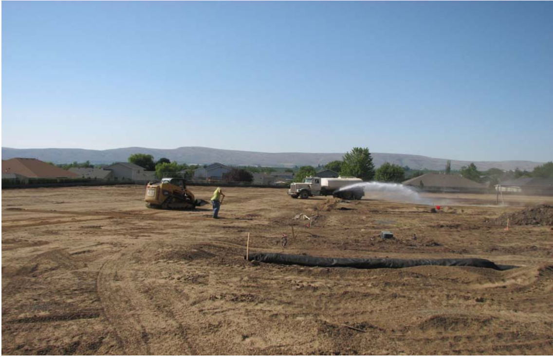
Photo D-1: Apple Valley Elementary School clean soil cap installation with dust control.
