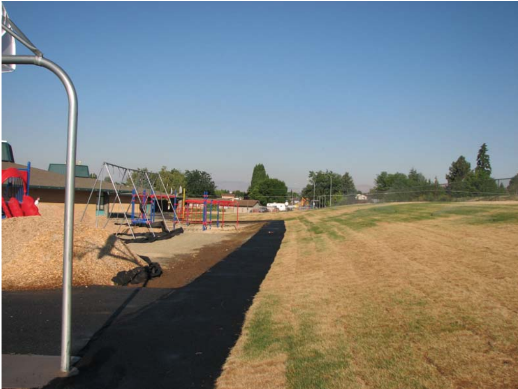
Photo D-6: Apple Valley Elementary School playground area construction.
