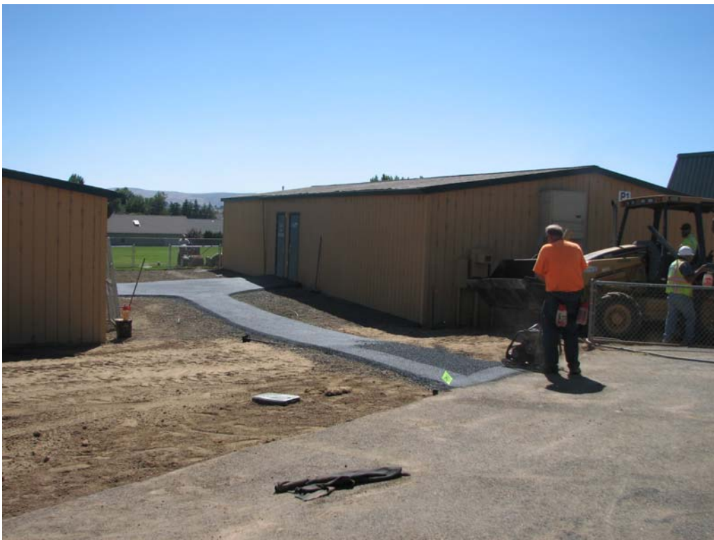
Photo D-4: Apple Valley Elementary School construction activities around portable classrooms.
