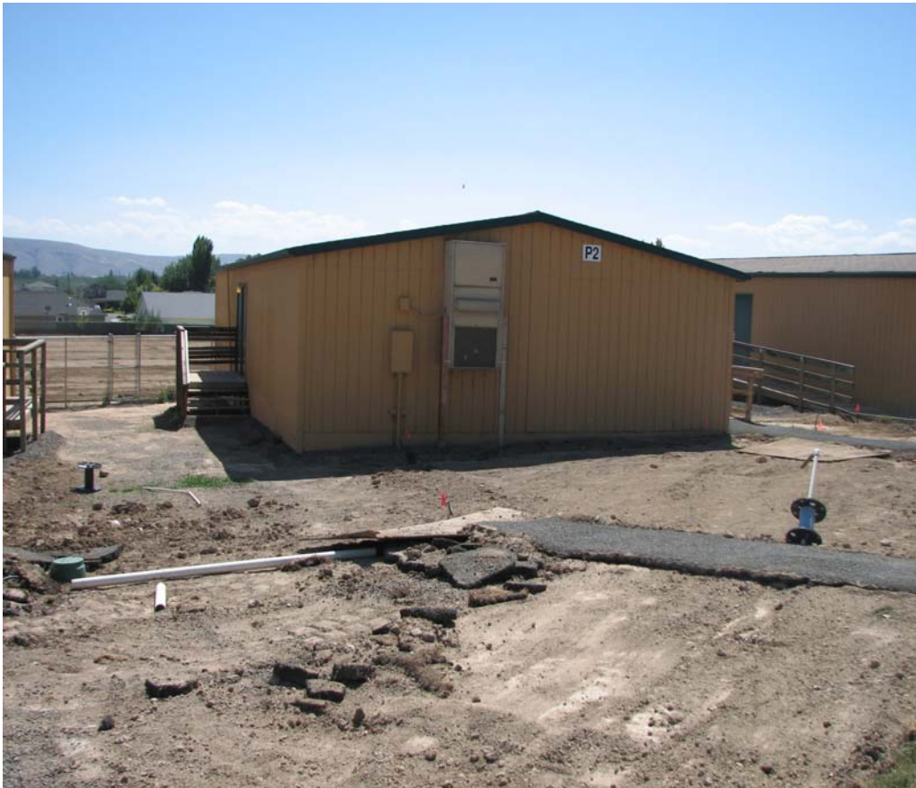
Photo D-3: Apple Valley Elementary School demolition activities around portable classrooms.
