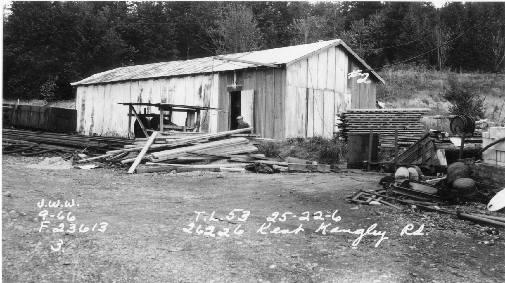
ROGERS #3 MINE SHOP (September, 1966; 252206-9053) This building housed machining tools, welders, parts and equipment for operating the Rogers #3 underground coal mine in Ravensdale. The entrance or portal to the mine is barely visible to the right of the photo. Located at 26226 Kent-Kangley Road under the BPA power lines, the Rogers #3 mine operated from 1963-1975 and produced 290,000 ton of clean coal.
