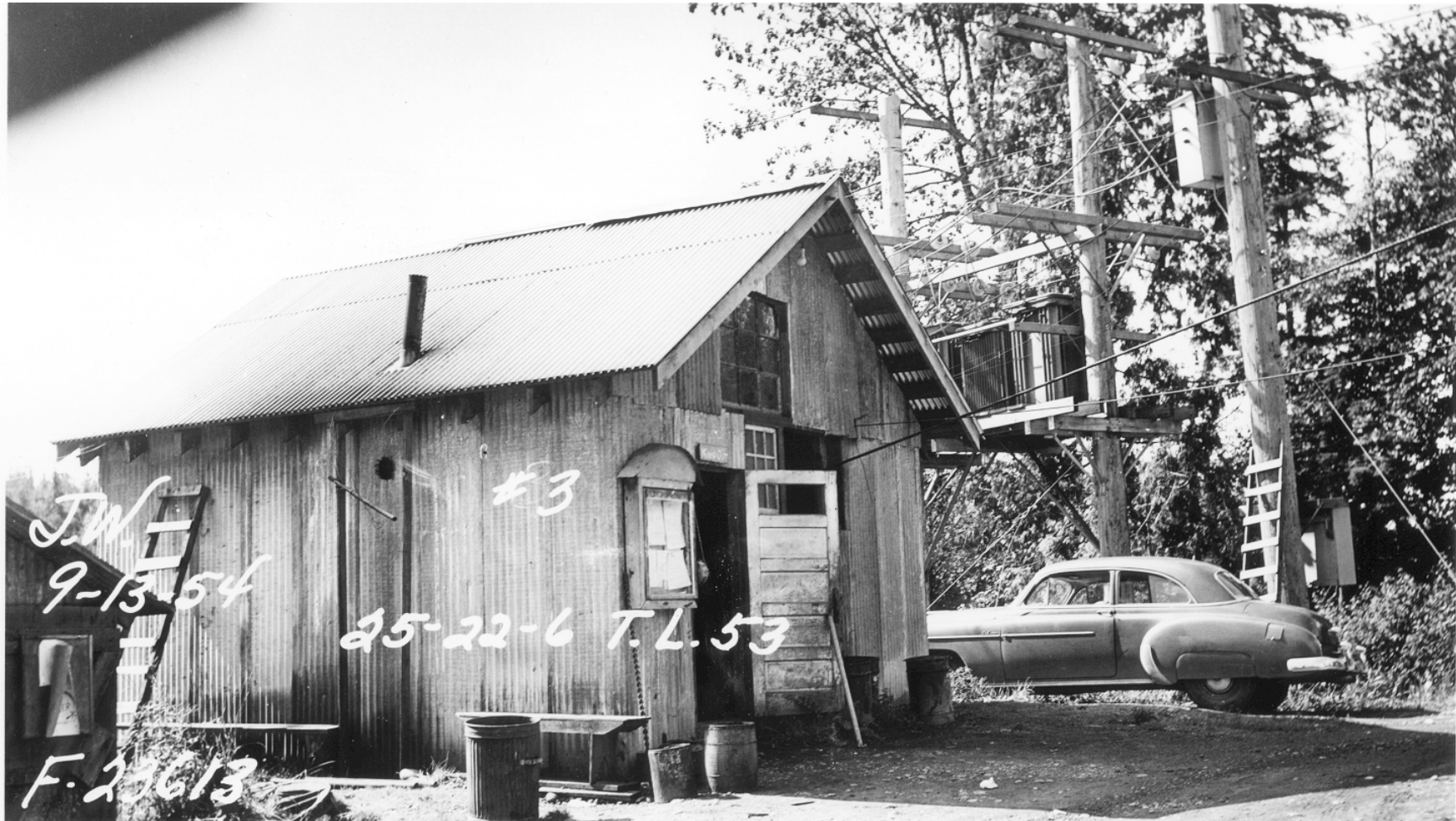
ROGERS #3 HOIST ROOM (circa 1966; #252206-9053) This building housed a large drum upon which a thick steel cable was spooled and unspooled as coal cars were hoisted up and down the steep slope carrying coal from up an underground slope which was over 600 feet deep. Located at 26226 Kent-Kangley Road, near Ravensdale, the Rogers #3 coal mine operated from 1963-1975 and produced 290,000 ton of clean coal.
