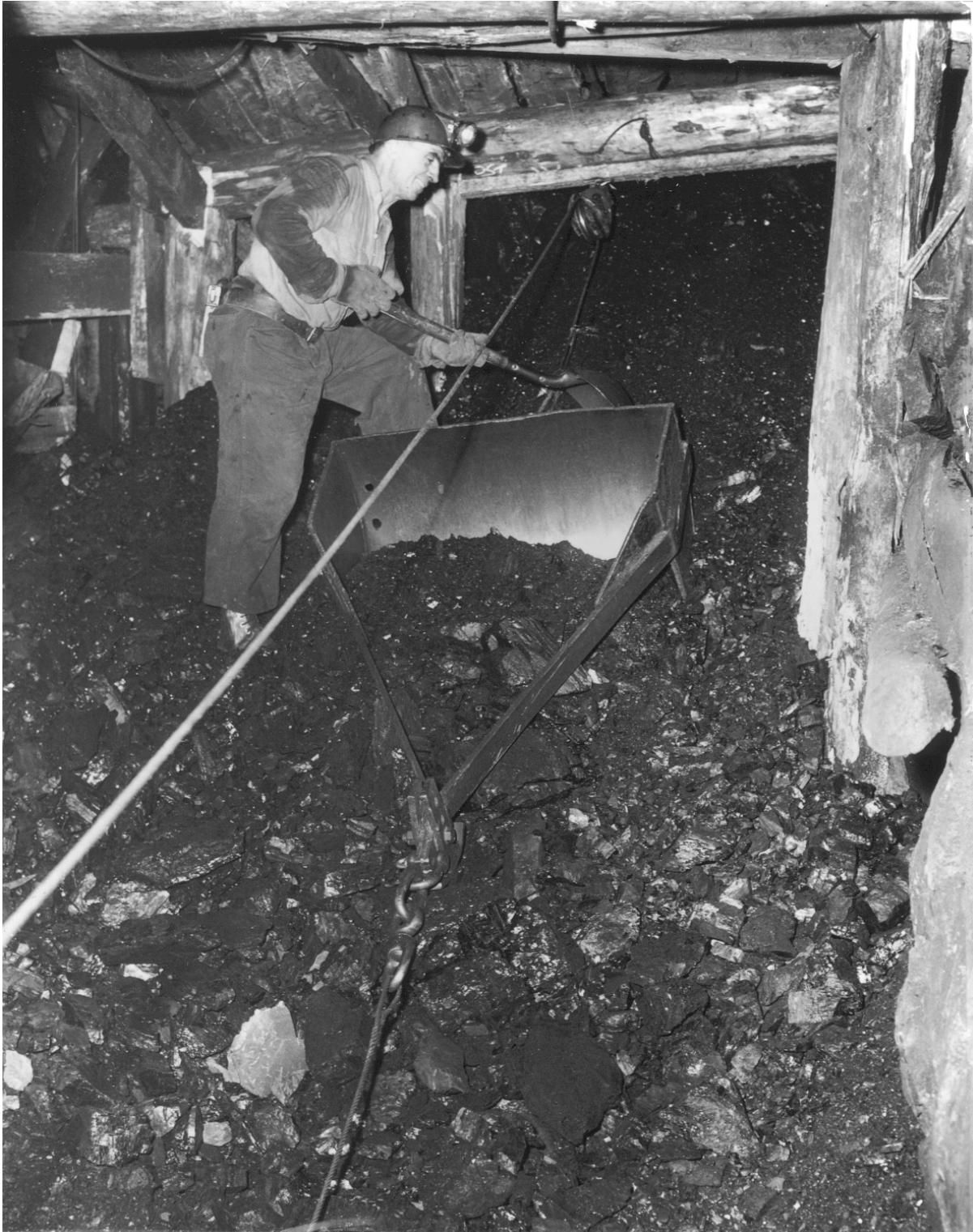
After a blast of dynamite, John Skulas of Maple Valley pulls the shattered coal with a large bucket guided by steel cables and powered by an electric winch. –Landsburg Mine, circa 1953. Photograph by the Seattle Times copyright 1978 Seattle Times P.O. Box 70, Seattle, WA 98111 all rights reserved; (206) 464-229.7 This picture has been purchased for personal use only and must not be published, reproduced, or used for advertising purposes without written permission from the Seattle Times.
