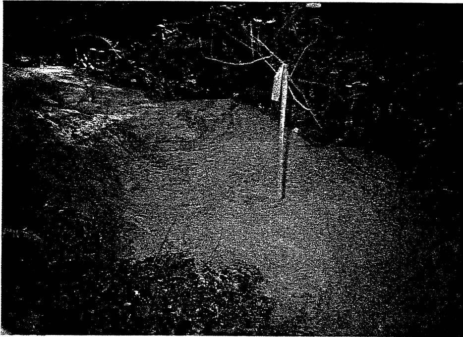
Photograph 7 - Completed CDF placement at L-01.
