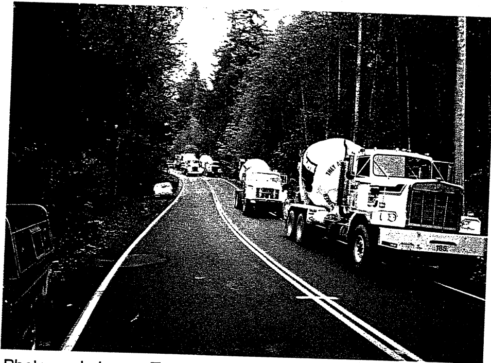
Photograph 1 - Trucks with CDF for L-01 backfilling.
