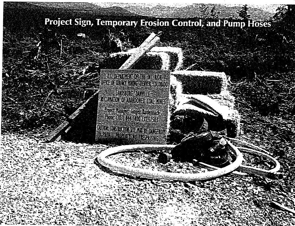
Photograph 1 Project sign, temporary erosion and sediment control, and dewatering hoses. Looking northeast. (WA-009_RV-01_082503a_Misc Equipment.jpg)
