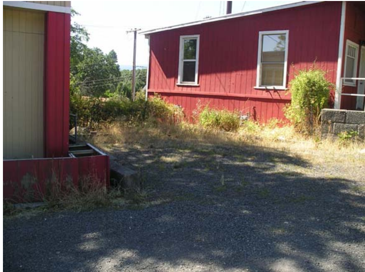
Photo 4: Space Between Former Station and Residence – from the east
