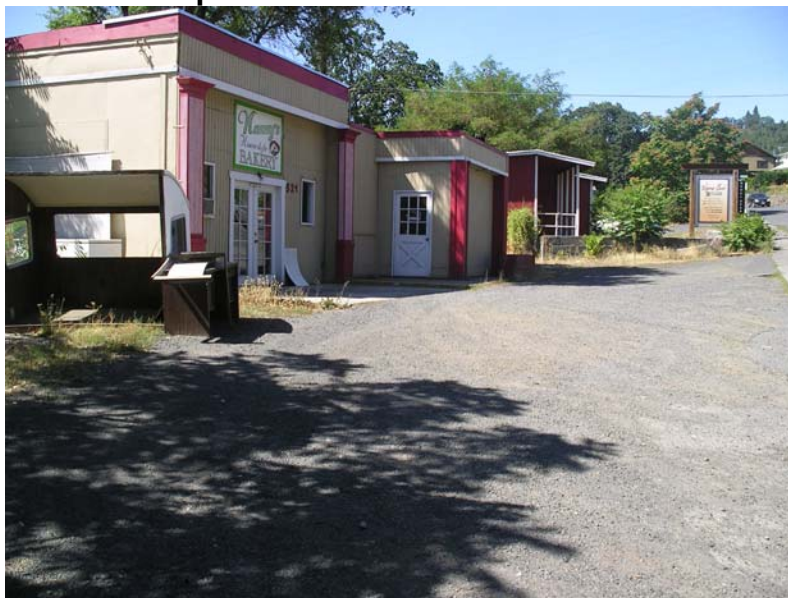
Photo 2: Former Town Pump Station - from the southeast
