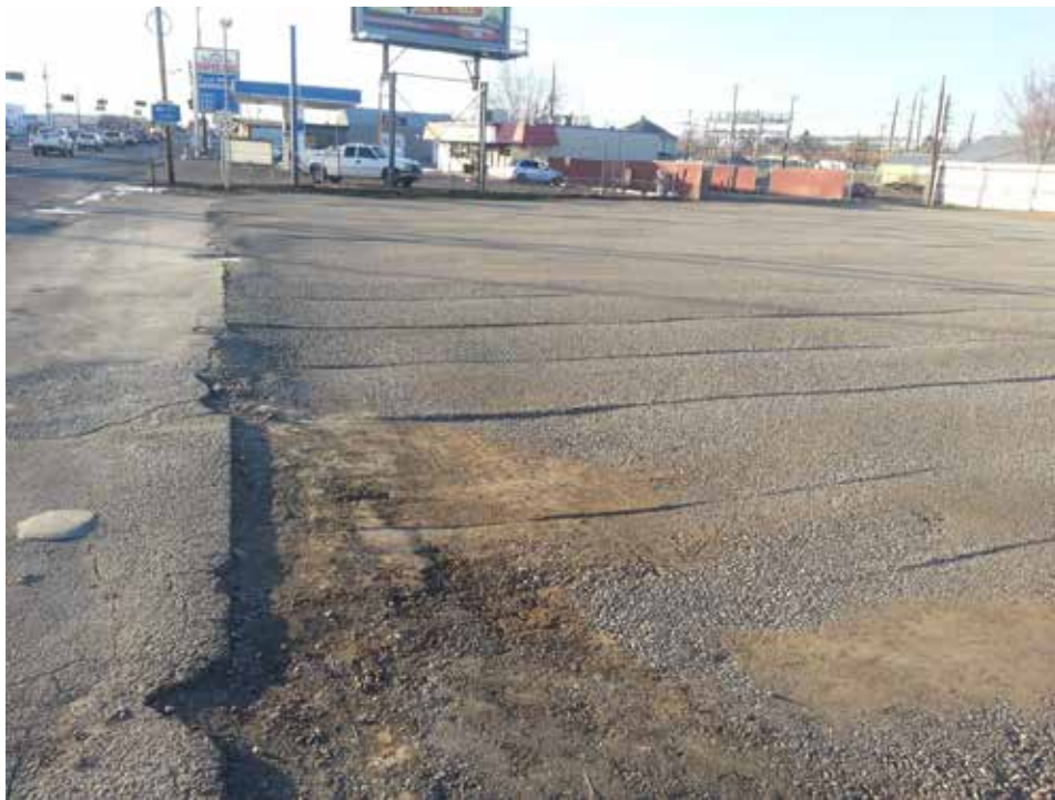
Photo 6: Trenching excavation along northwest road
