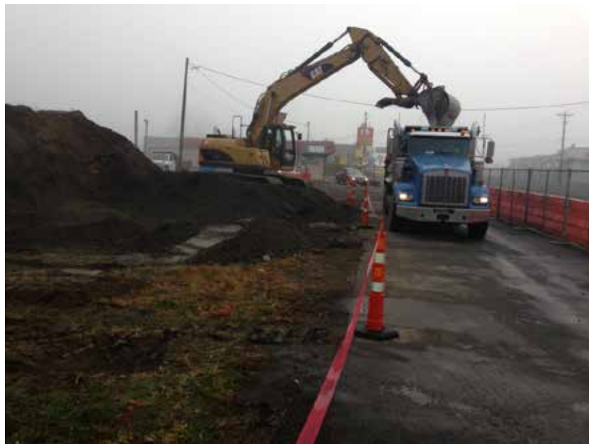
Photo 2: Loading trucks along southern property boundary for transport to disposal facility (11/12/2013)
