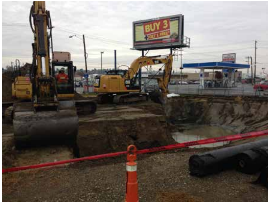
Photo 1: Excavating in northwest corner of site (11/12/2013).
