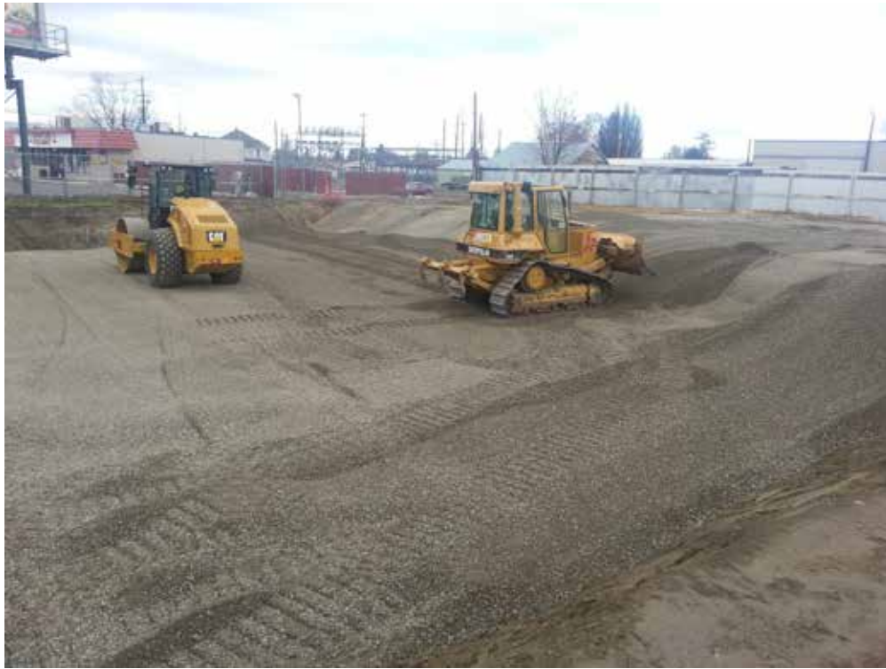
Photo 5: Trenching excavation along northwest road (11/19/2013).
