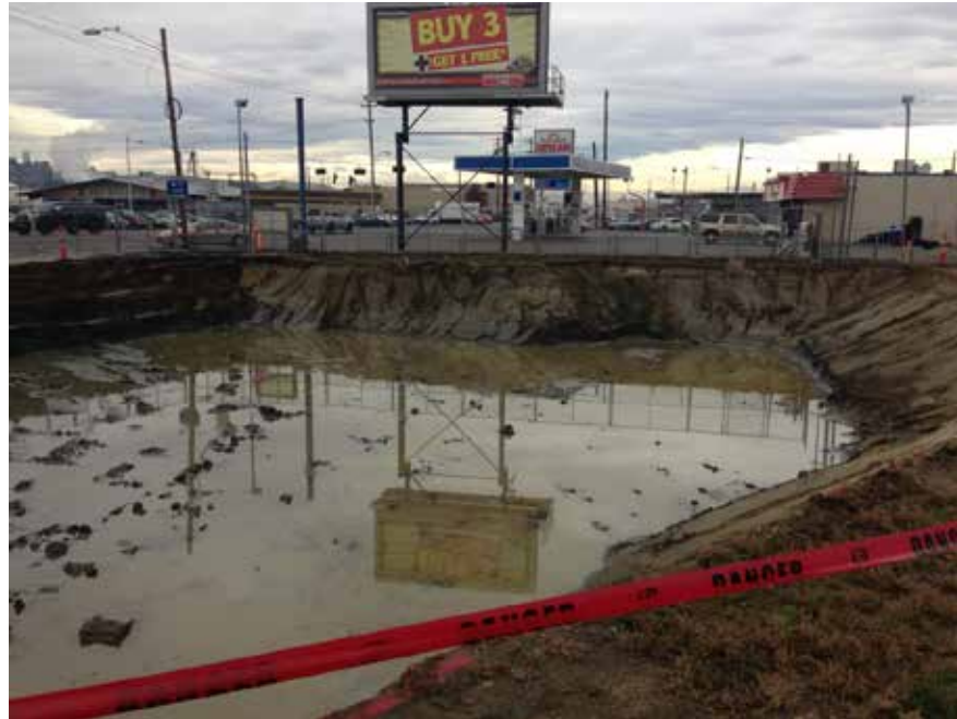
Photo 3: Complete open excavation prior to backfill (11/15/2013).
