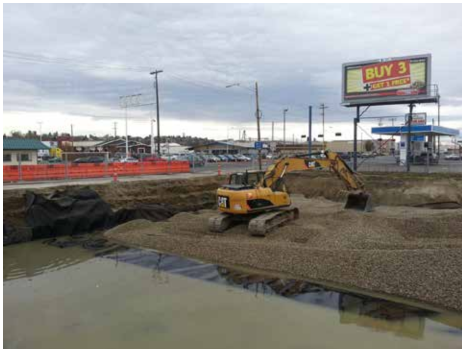
Photo 4: Excavator placing gravel over Geotextile on base of excavation (11/18/2013).
