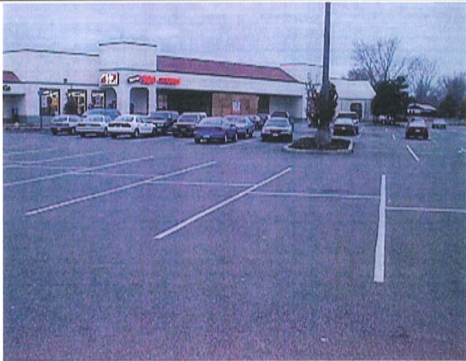
Photo 3: View looking southwest across the Site parking lot toward Flaherty's 99 cent Store (former Ernst).
