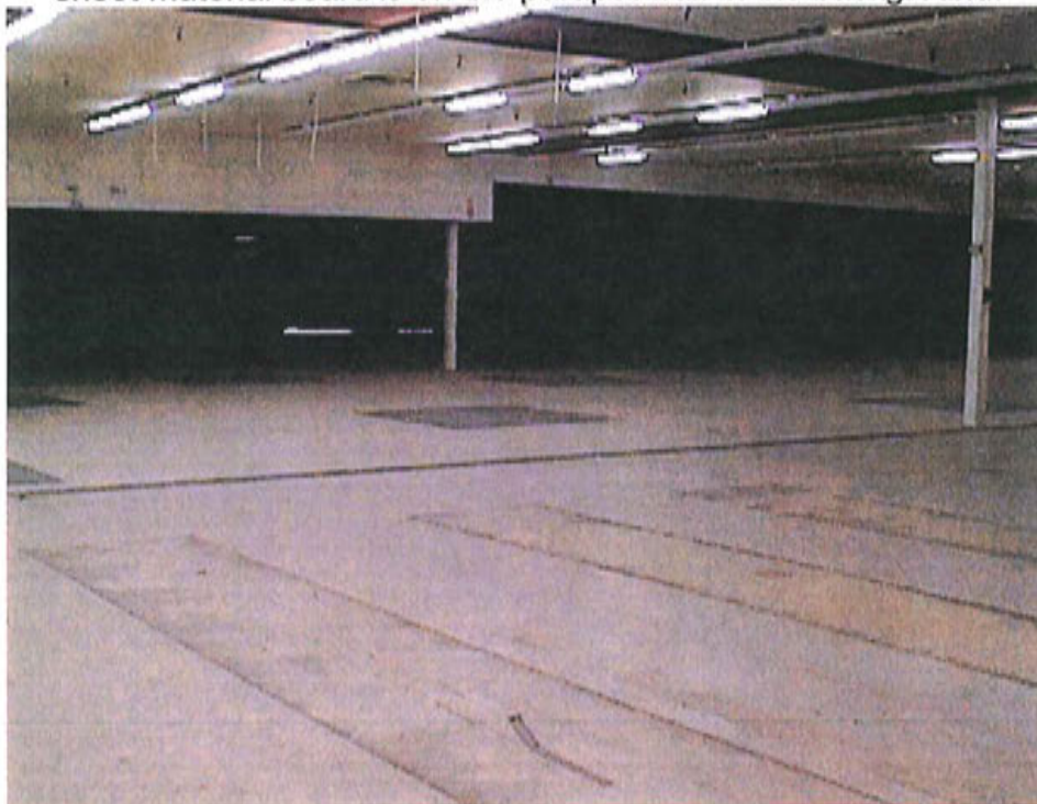
Photo 10: View of the interior of the former Ernst store. Asbestos-containing floor tile mastic is beneath the floor tiles.
