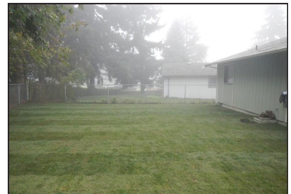
We install sod to replace the lawn.
