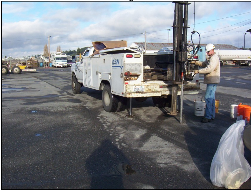
Boring #7. UST nest to left of probe rig.
