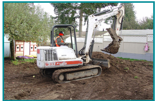
Cleanup involves soil removal, replacement, and re-landscaping
