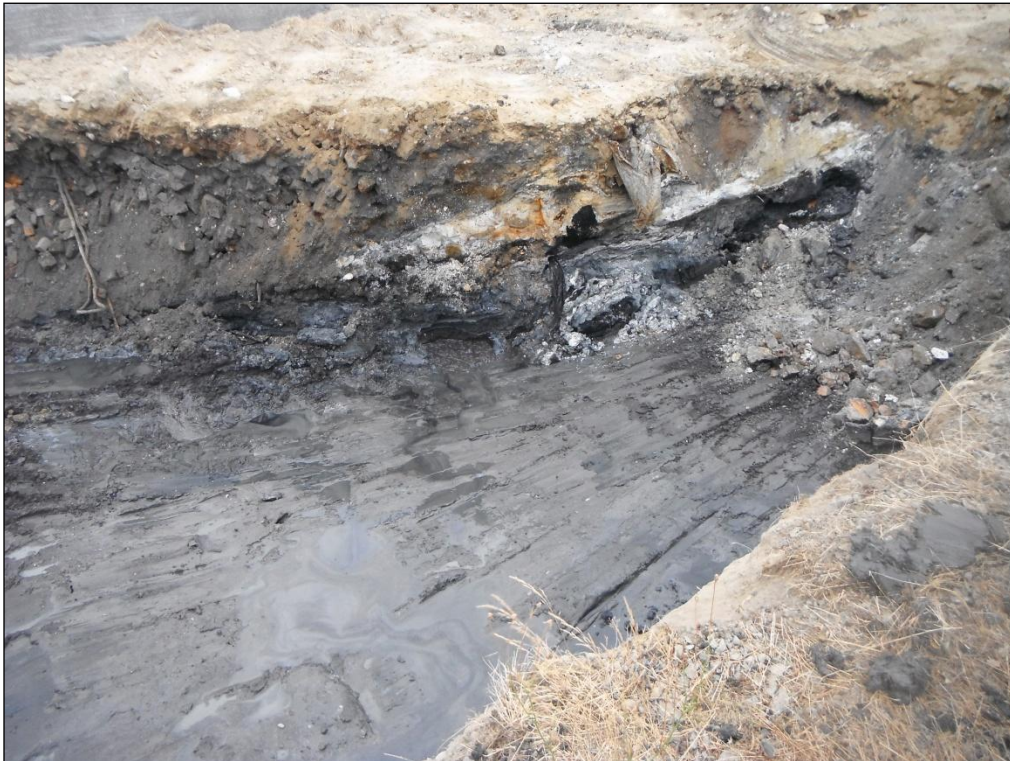
4. Closed Landfill waste and underlying native silty material.
