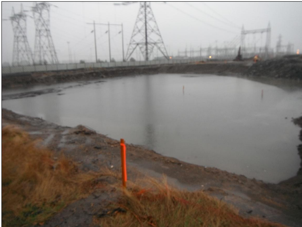
6. Looking southwest across the completed Closed Landfill excavation after a rise in groundwater level.
