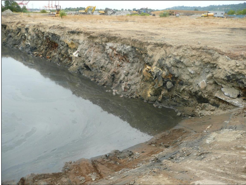
3. Representative waste material excavated from the Closed Landfill area, including bricks, concrete fragments, rebar, plastic sheeting, etc.
