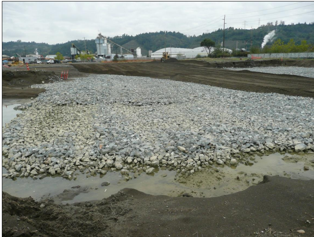
7. Looking north across the Closed Landfill area after placement of quarry spalls and during placement of surficial sand fill material.
