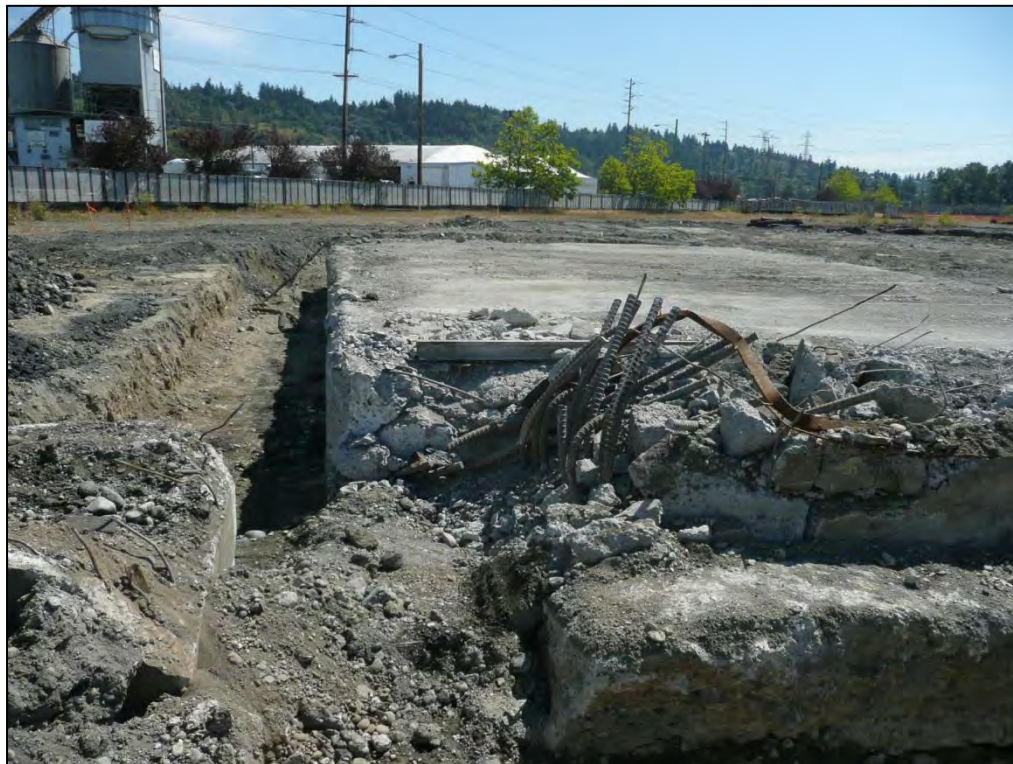
8. Close-up view of heavy rebar and steel rail reinforcement in the pot dumping slab.
