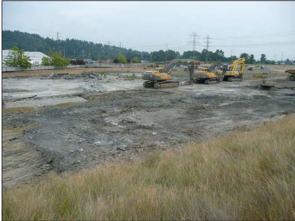
3. Looking southeast across the SPL Area during demolition of surficial concrete slabs and asphalt pavement.
