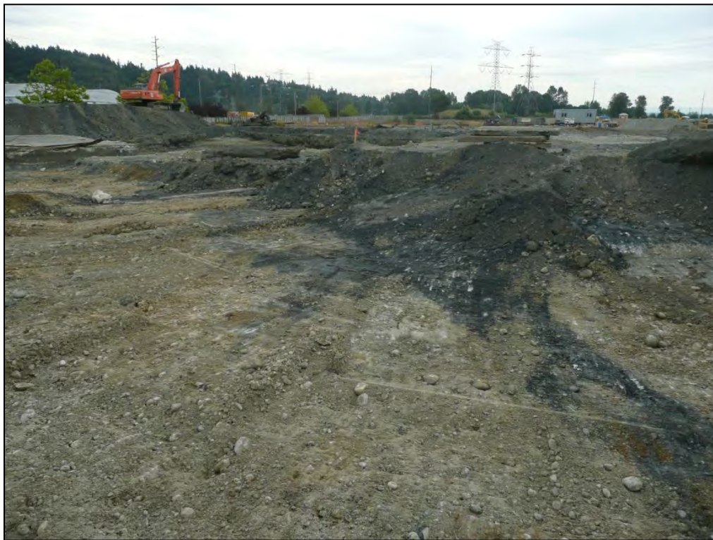
6. SPL zone material (dark gray) and underlying uncontaminated soil.
