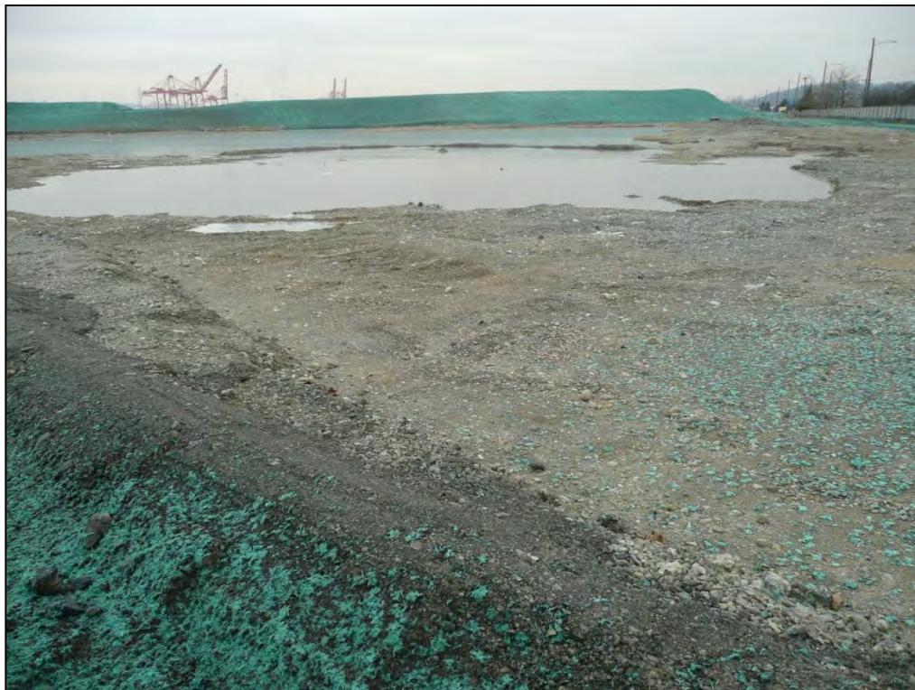
18. Looking northwest across the completed SPL Area excavation toward the dredged soil stockpile, with water ponded in a significant portion of the excavation.
