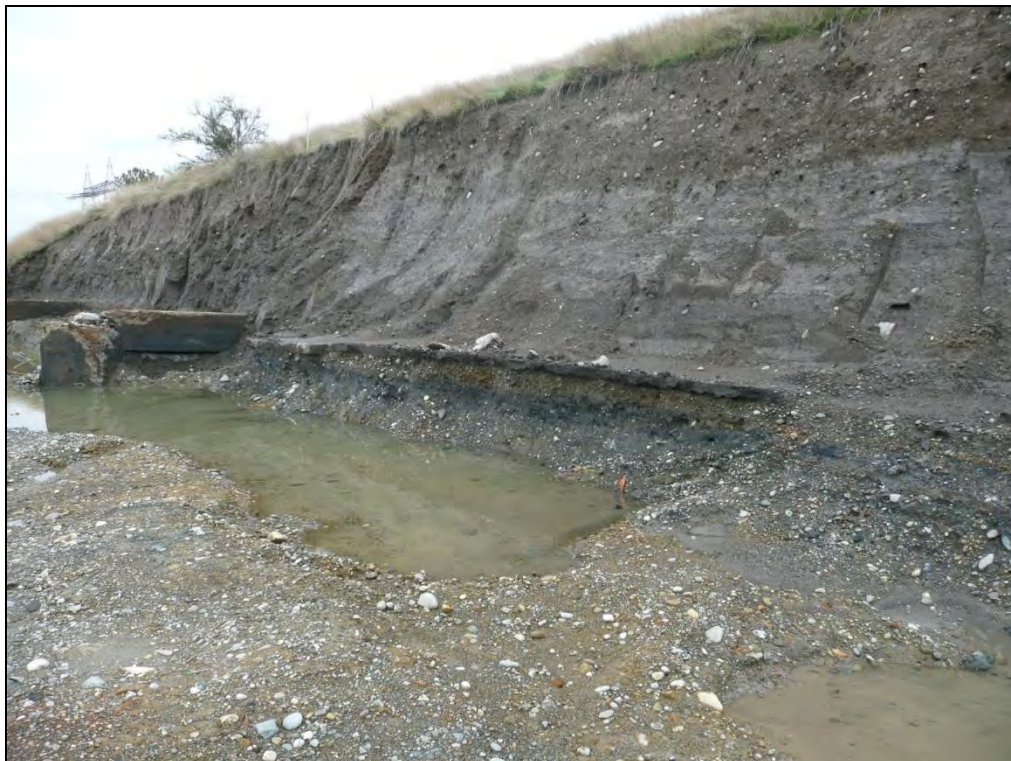
12. Looking southwest at a layer of SPL material extending under the dredged soil stockpile.
