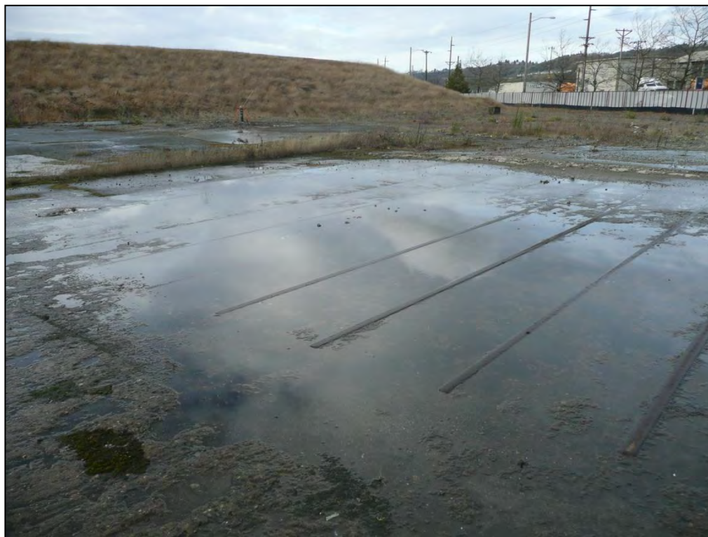
2. Looking northwest across the steel rails embedded in the surface of the pot dumping slab in the former SPL management facility.
