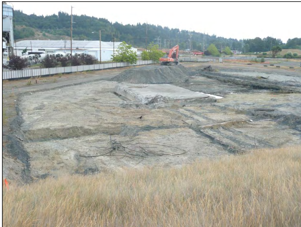
10. Looking southeast across the SPL Area excavation, with view of pot dumping slab, SPL material in utility trenches, and temporary stockpile of excavated SPL material to be loaded for disposal.
