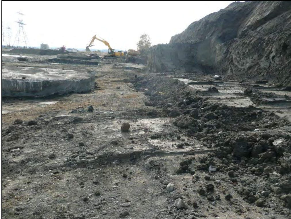
13. Looking south along the west side of the foundations of former buildings exposed during SPL material removal under the dredged soil stockpile.
