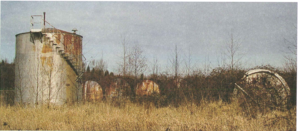
Treoil4a: Abandoned ASTs at the site. Tanks in the background are also visible in Treoil1. The rosin pile in Treoil1 is just north of the background tanks. This photo is a cropped version of Treoil4. View is to the north. The north side of the site chain link fence is visible between the tanks in the foreground and the background tanks.
