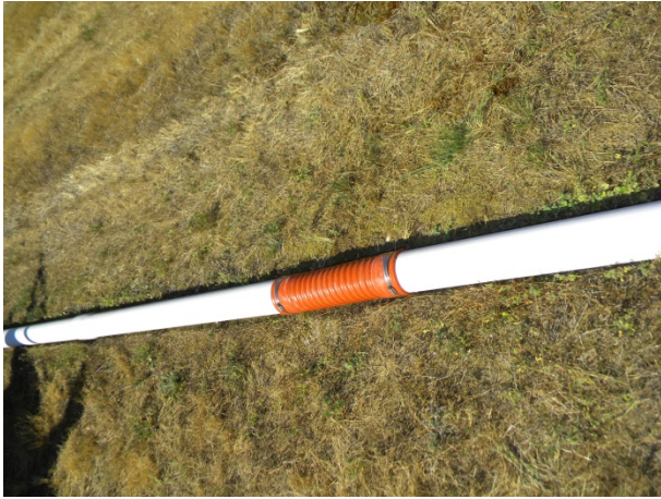
E-40. Replaced damaged 4-inch landfill gas flex hose.
