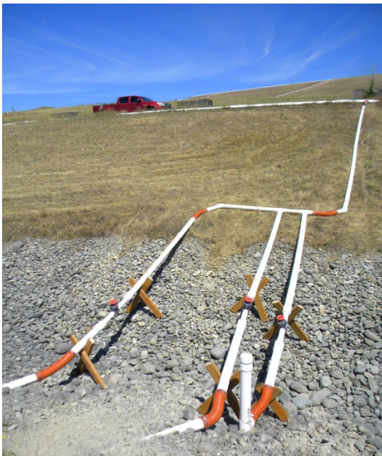
N-64A, N64B, and N64C. Replaced damaged 3-inch gate valves and damaged landfill gas flex hoses and installed risers to re-grade drainage for gas wells.
