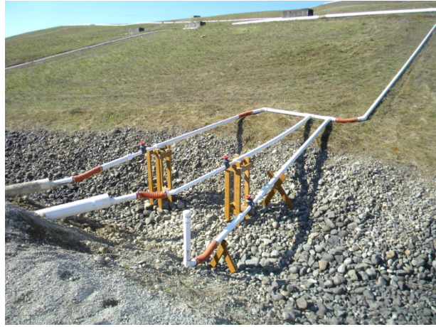
N-64B and N-64C. Pipe supports north of the perimeter road to improve drainage.
