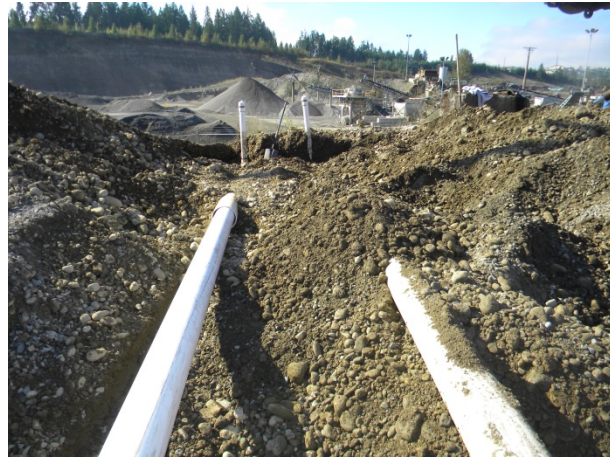
N-64B and N-64C. Re-grading of lateral piping to improve drainage.
