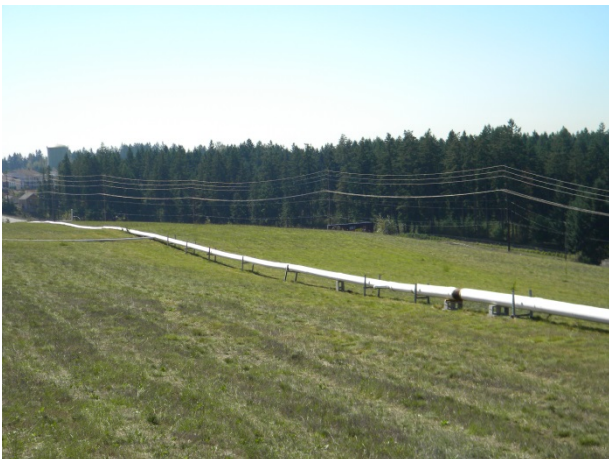
N-64B and N-64C. LFG header pipe along the southwest crown of the landfill that requires additional slope adjustment.
