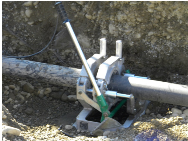
Leachate Force Main. Repaired damage to 4-inch diameter leachate force main.
