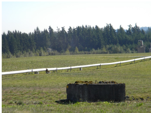
N-64B and N-64C. LFG header pipe along the southwest crown of the landfill that requires additional slope adjustment.
