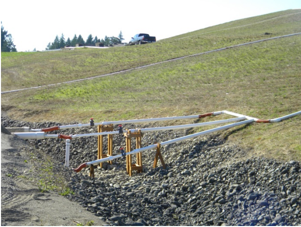
N-64B and N-64C. Pipe supports north of the perimeter road to improve drainage.
