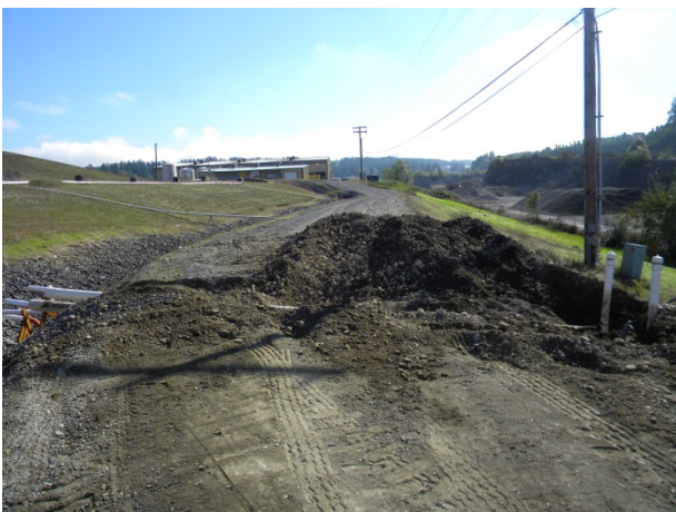
N-64B and N-64C. Trenching across the perimeter road, and final completion.
