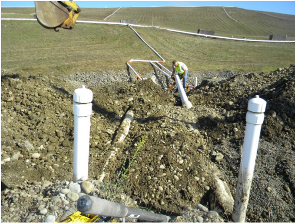
N-64B and N-64C. Re-grading of lateral piping to improve drainage.
