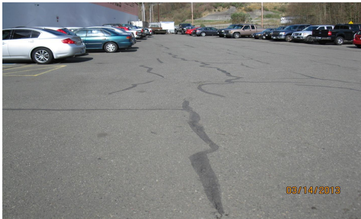
Photo 8: Patched/Repaired Asphalt Cap – From Southeast
