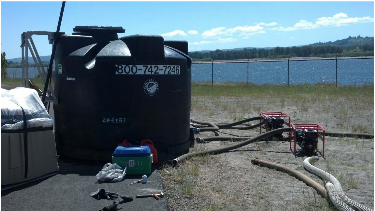
Photograph 2: Injection equipment and materials
