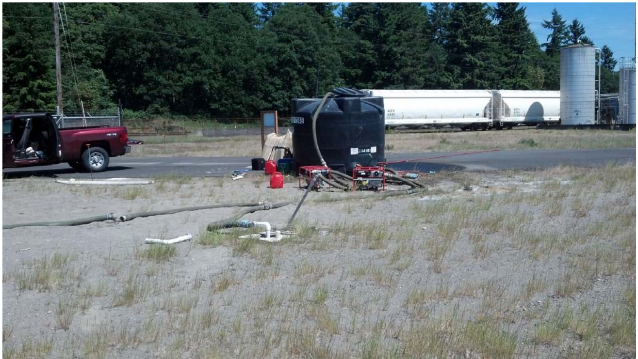
Photograph 4: Injection into IW-12
