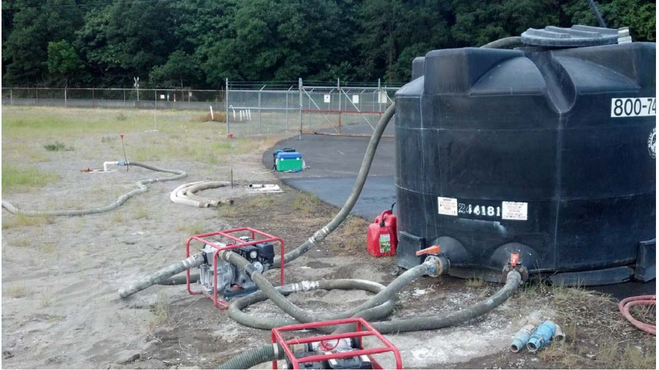
Photograph 3: Injection into IW-8
