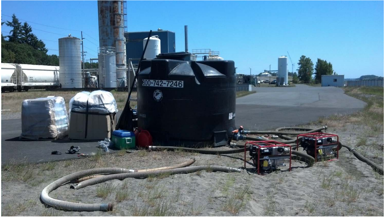
Photograph 1: Injection equipment and materials
