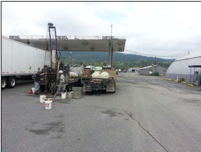
Figure 1. Exploration Activities at Borehole 1
