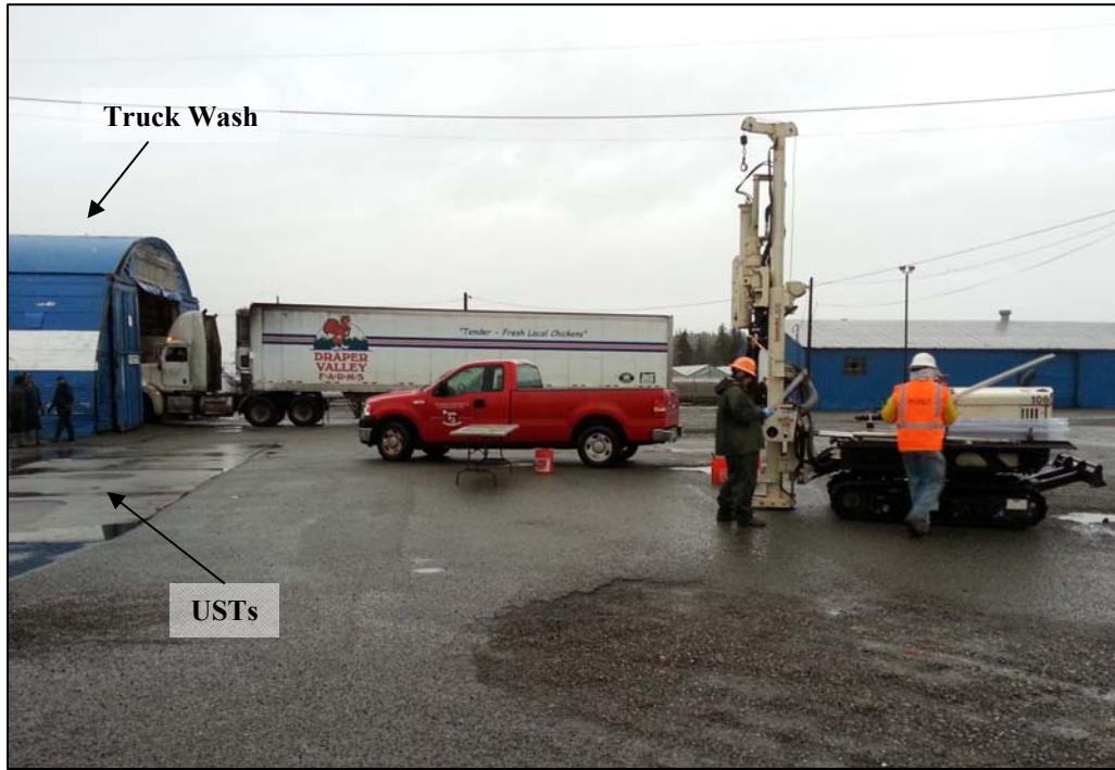
Photo 1. Borehole B-1 in progress. Existing USTs to left. Looking North.
