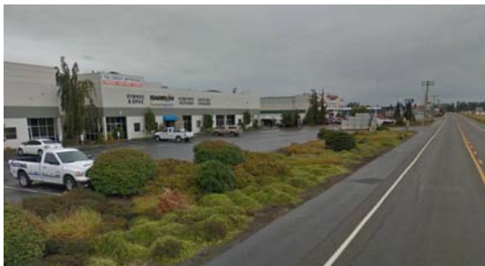
A variety of commercial and industrial uses are located in the south Mount Vernon area.
