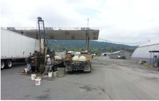
Geotechnical exploration activities at the Truck City Site.
