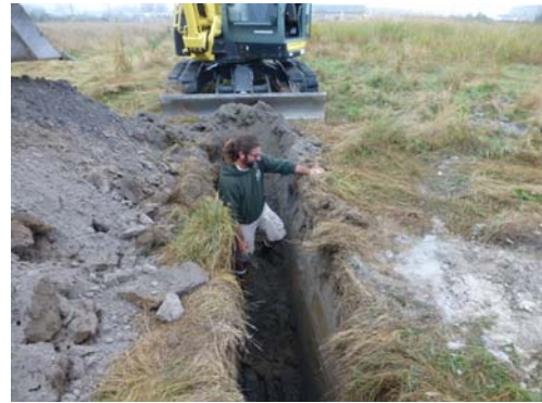
Trench excavations at the Alf Christianson Seed Site
