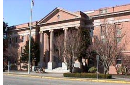
The area surrounding the site includes a variety of public/civic uses, such as the County Courthouse.
