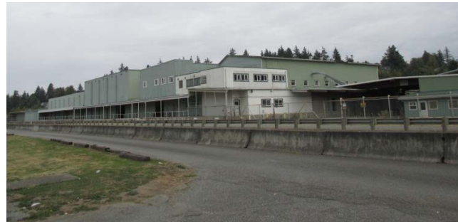
Vacant seed processing buildings on the Alf Christianson Seed Site.
