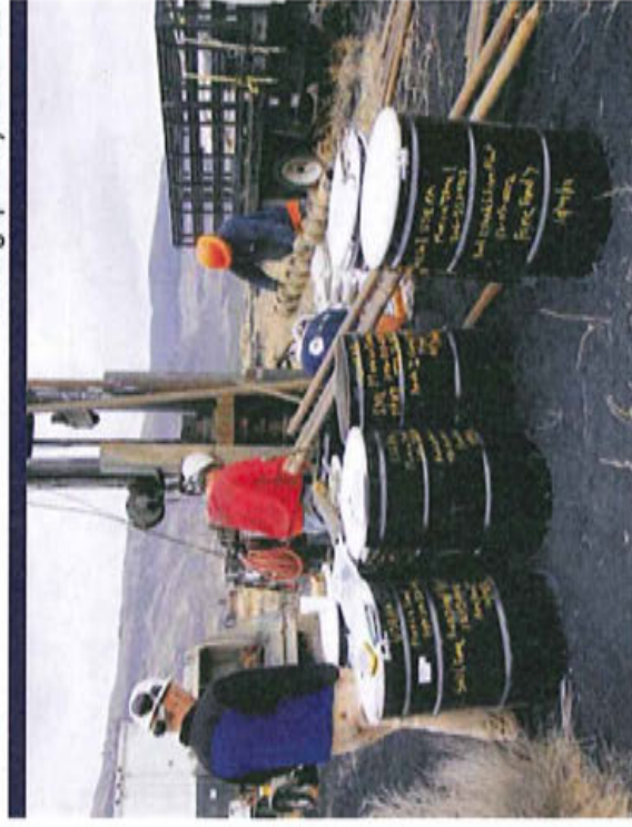
Photo 14 Investigation-derived waste drums from FP07. Seven drums of soil cuttings. All are labeled.
