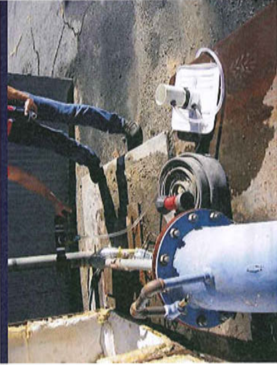
Photo 1 Wellhead of production well No. 2.
