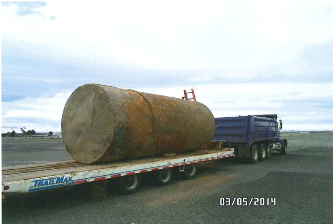
6000 GALLON UST SECURED FOR TRANSPORT
