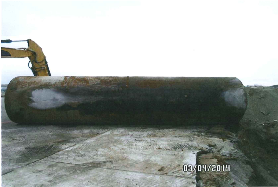
12000 GALLON UST AFTER REMOVAL
