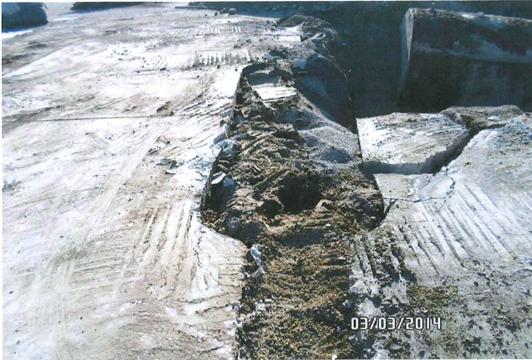
REMOVED PUMP ISLAND
