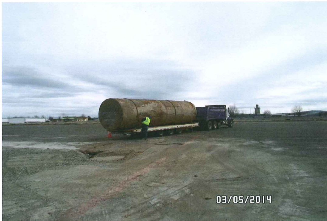
12000 GALLON UST SECURED FOR TRANSPORT
