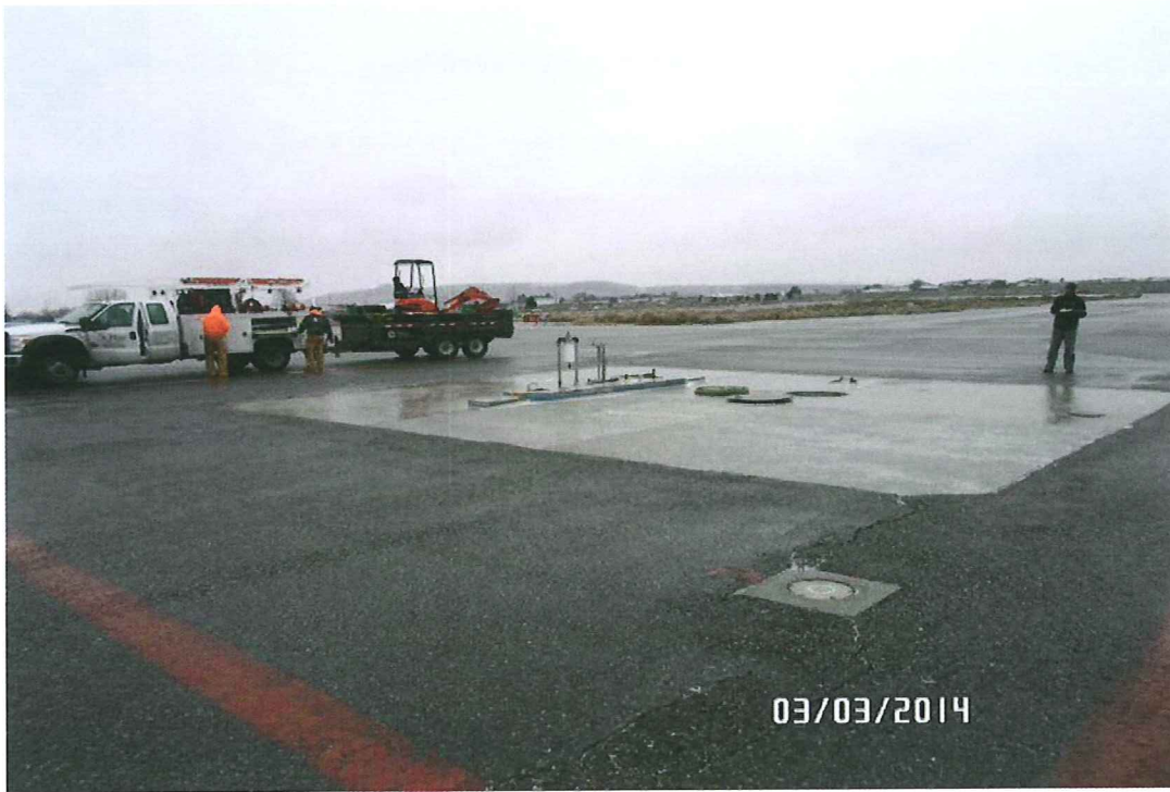
SITE PRIOR TO EXCAVATION
