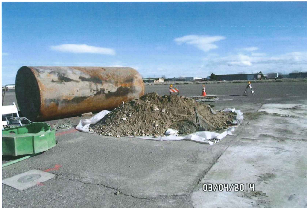
6000 GALLON UST AFTER REMOVAL AND STOCKPILED SOIL
