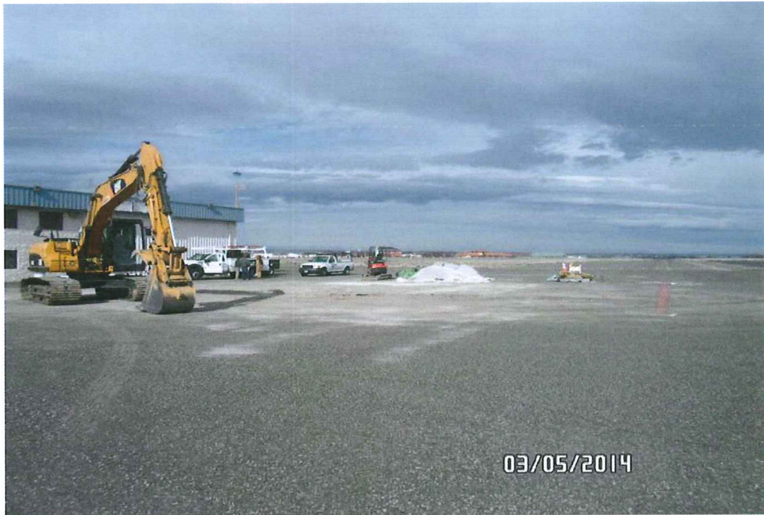
SITE AFTER BACKFILLING AND UST REMOVAL
