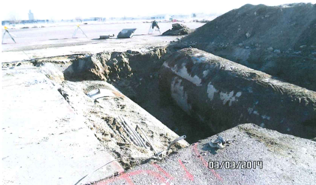
EXCAVATION OF USTs
