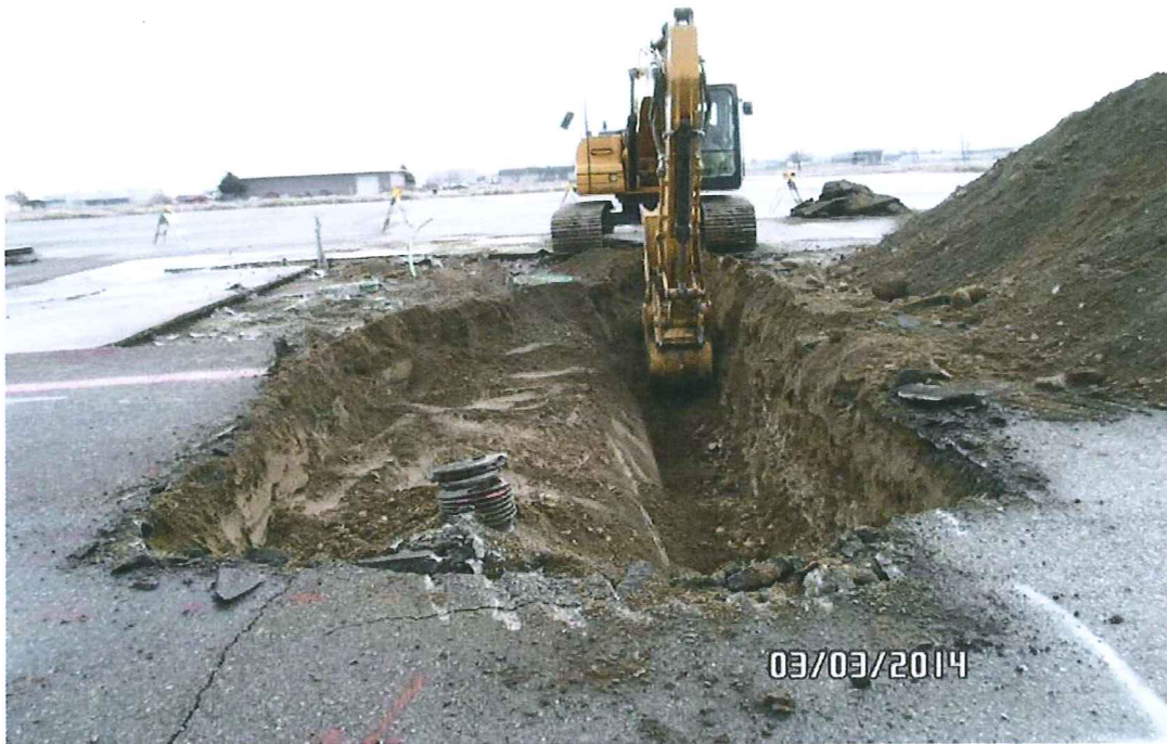
EXCAVATION OF USTs.
