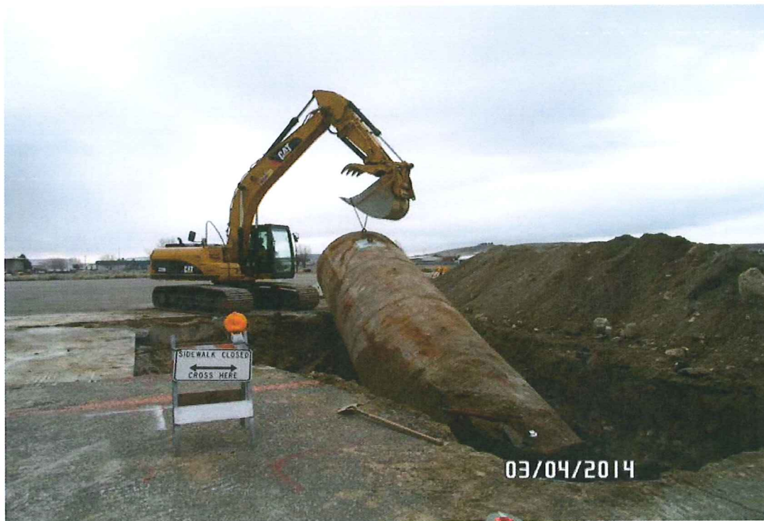
REMOVAL OF 12000 GALLON UST
