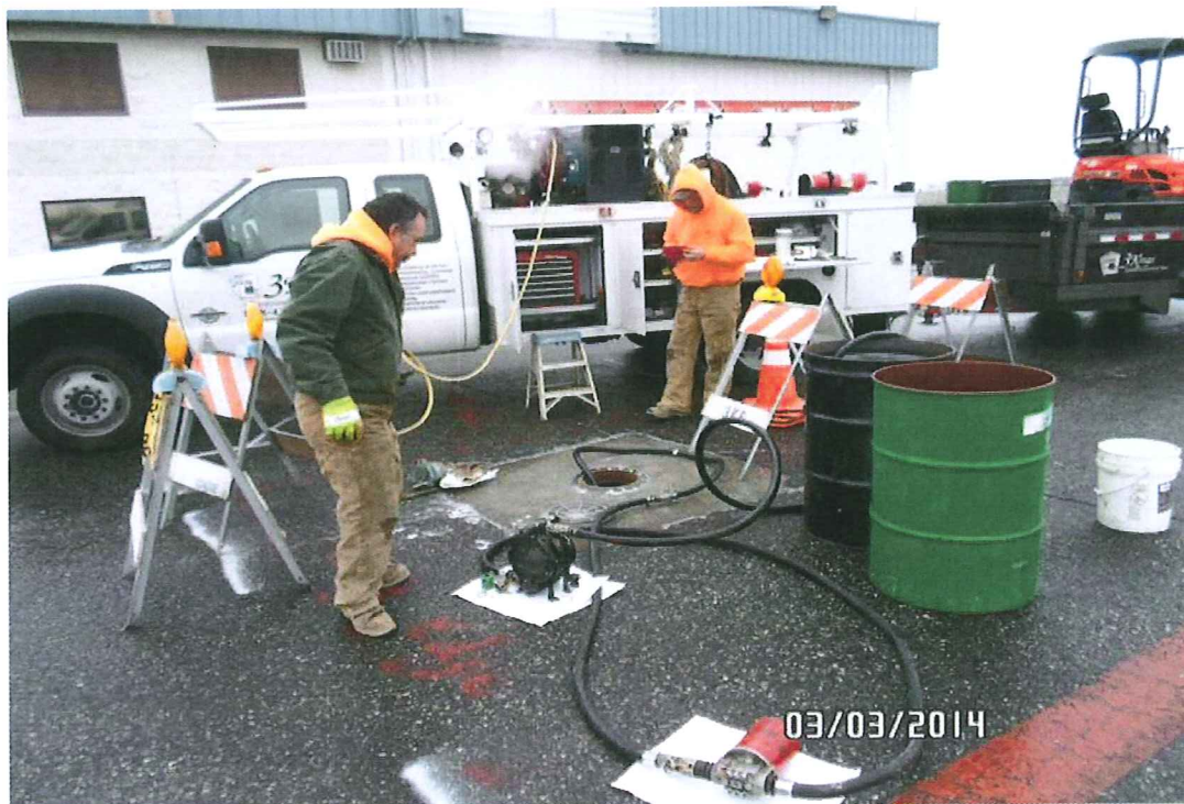
REMOVING RESIDUAL FUEL
