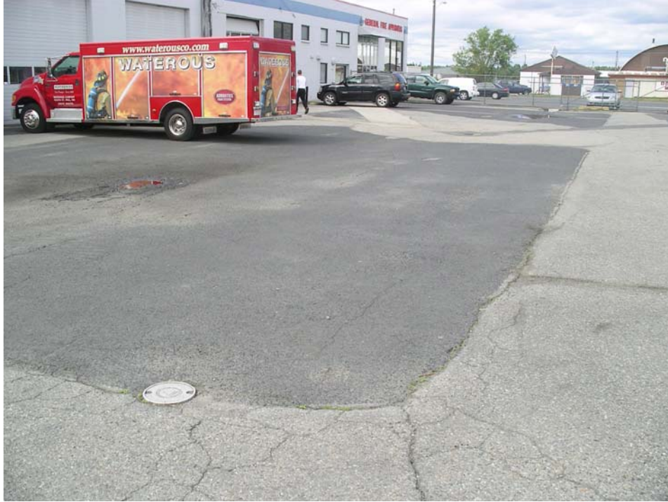
Photo 3: North Side of Building - from the southeast
