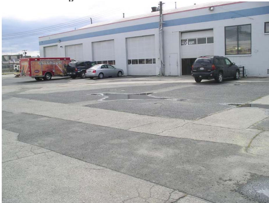
Photo 2: East Side of building - from the northeast
