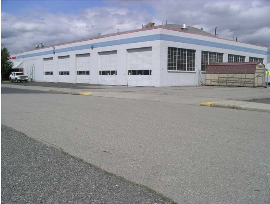
Photo 1: Southwest corner of the building - from the southwest
