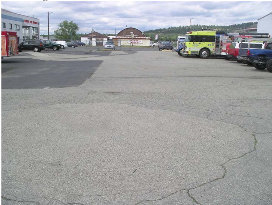
Photo 4: West Parking Area – from the south
