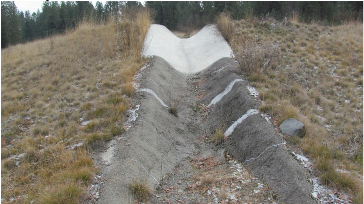
Photo 2: Repaired Concrete Drain Channel - from the northwest
