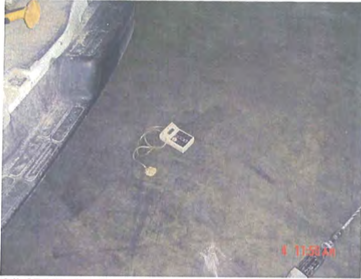
6-4-07 VIMS-1 Puget Sound Pipe Warehouse– Shows Digital Micromanometer recording the negative pressure differential over a test hole
