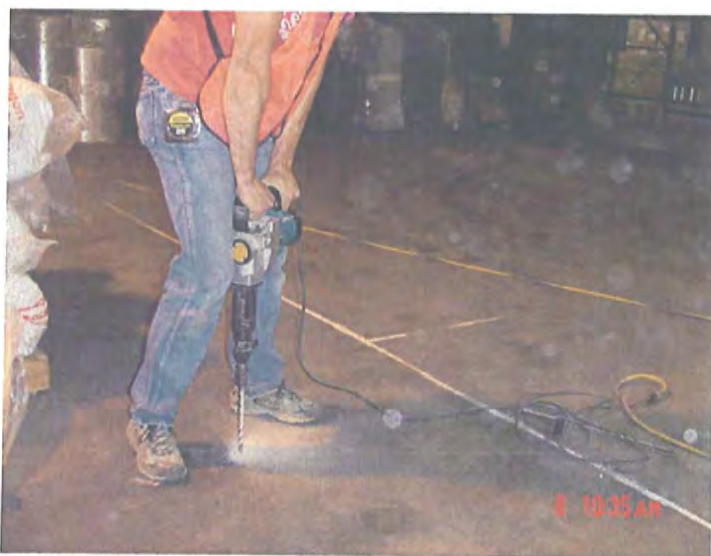
6-6-07 VIMS-3 Hudson Bay Warehouse (Facing North) – ART contractor drilling TH-8
