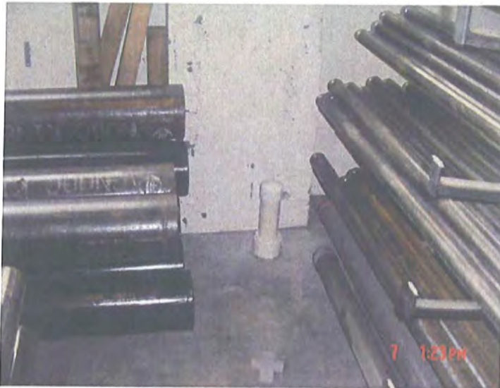
6-7-07 VIMS-1 Puget Sound Pipe (Facing North) – Capped Riser after excavation of sump
