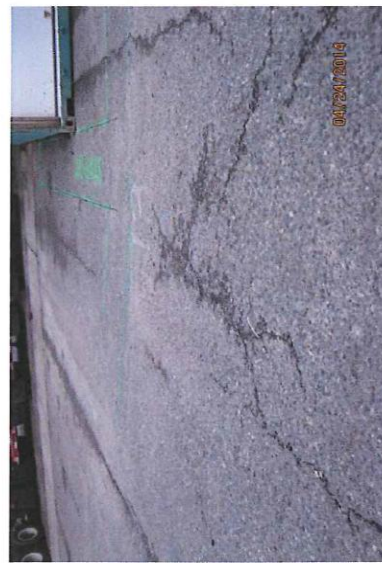
Photo 7: Small Cracks in the Asphalt Cap
