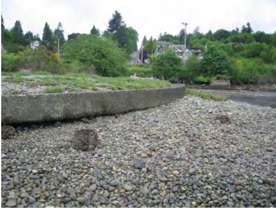
Photo 5 Beach and intertidal substrate sizes and concrete wall, looking north
