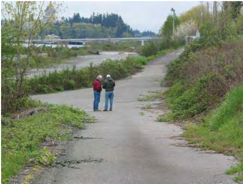
Photo 1 Overview of upland area, looking south; invasive vegetation and concrete roads/pads are visible in the foreground and upper left
