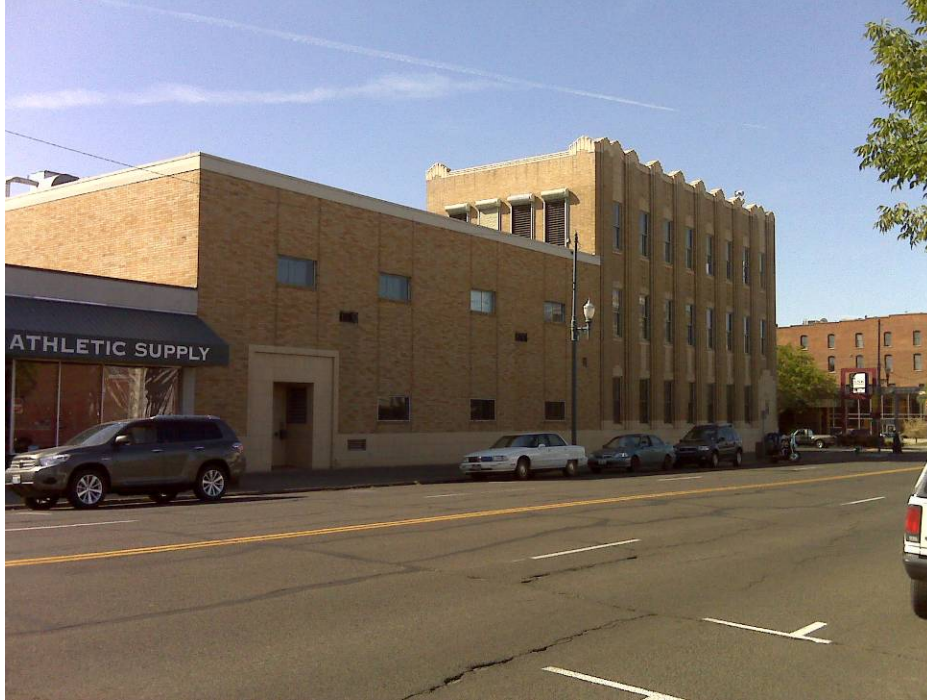
Photo 1: US West Building - from the northeast
