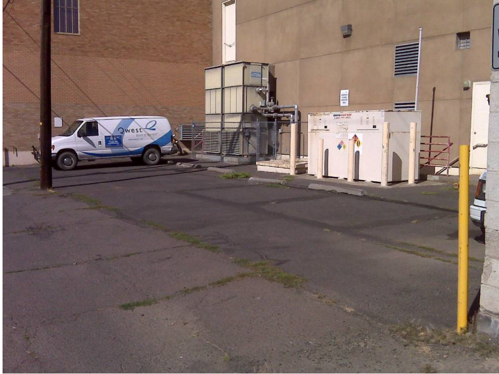
Photo 3: Former UST Location - from the east
