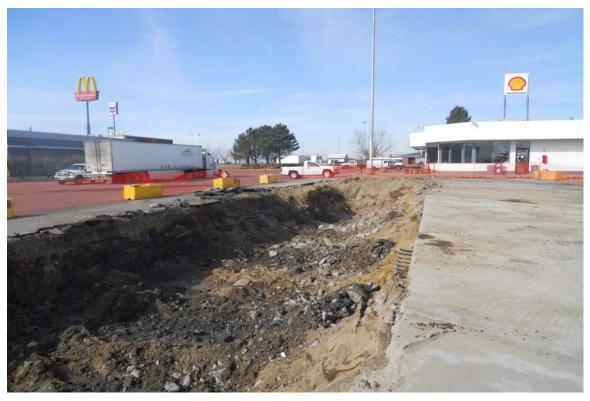
EXCAVATION AFTER FOUNDATION REMOVAL
