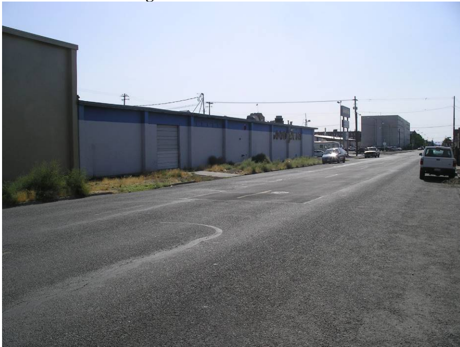
Photo 4: West Side of the Building – from the northwest
