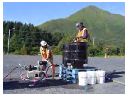
RegenOx Soil Mixing Application
