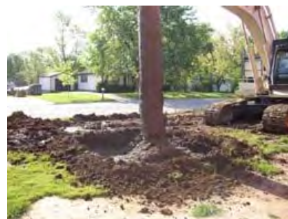
Post-Injection RegenOx Field Setup RegenOx Soil Mixing Application Field Operations Injection Setup
