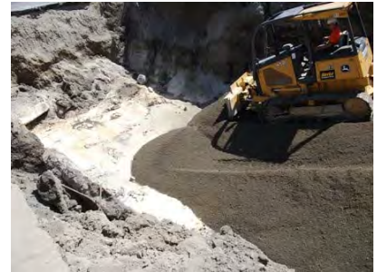
Type 17 Being Placed Over Top Of ORC /Oxygen Release Compound
