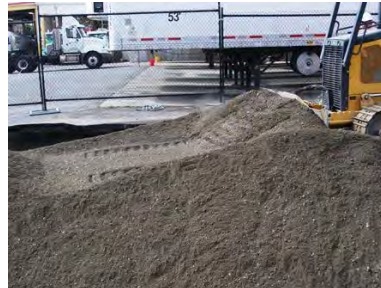
Type 17 Material being Pushed Stockpile / South View
