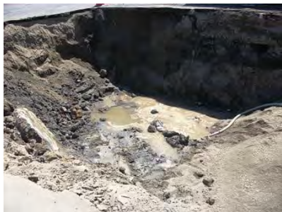
Water From Existing Storm Drain At Bottom Grade Elevation
