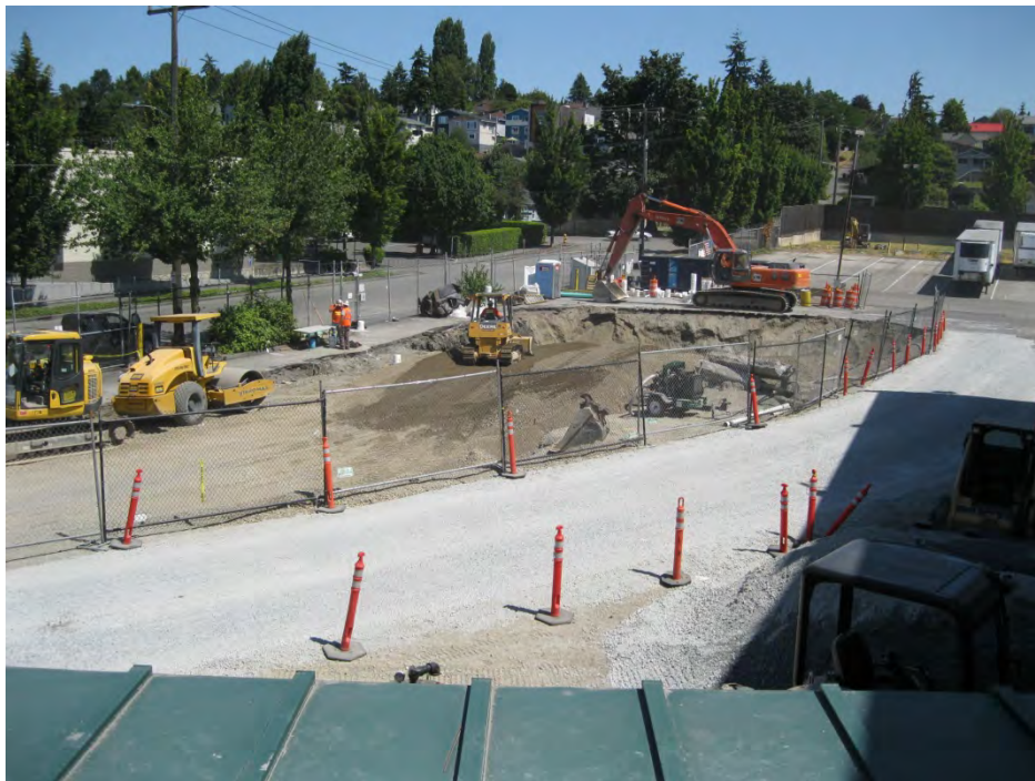
Photo 10: Backfilling and Compaction in Northeast Corner of Excavation, 8/4/2011
