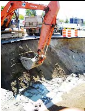
Next area of excavation 12 ft below
