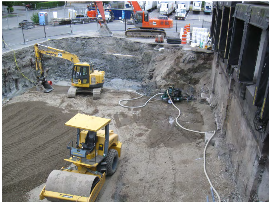
Photo 6: Excavation Backfilling and Compaction, with Dewatering Pump, 7/21/2011
