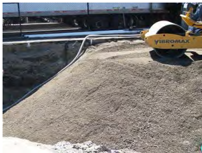
Type 17 Being Compacted @ 00+10 Grid / South View
