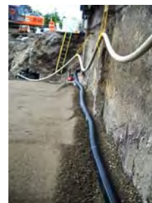
Drain pipe connected to existing Drain at 8ft level
