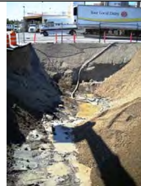
de-watering area before back-fill
