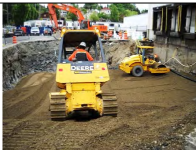
Ramp built to push-out each lift
