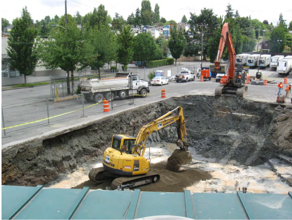
Photo 5: Start of Backfilling Activities (Note Regenesis Products Spread on Excavation Bottom), 7/20/2011
