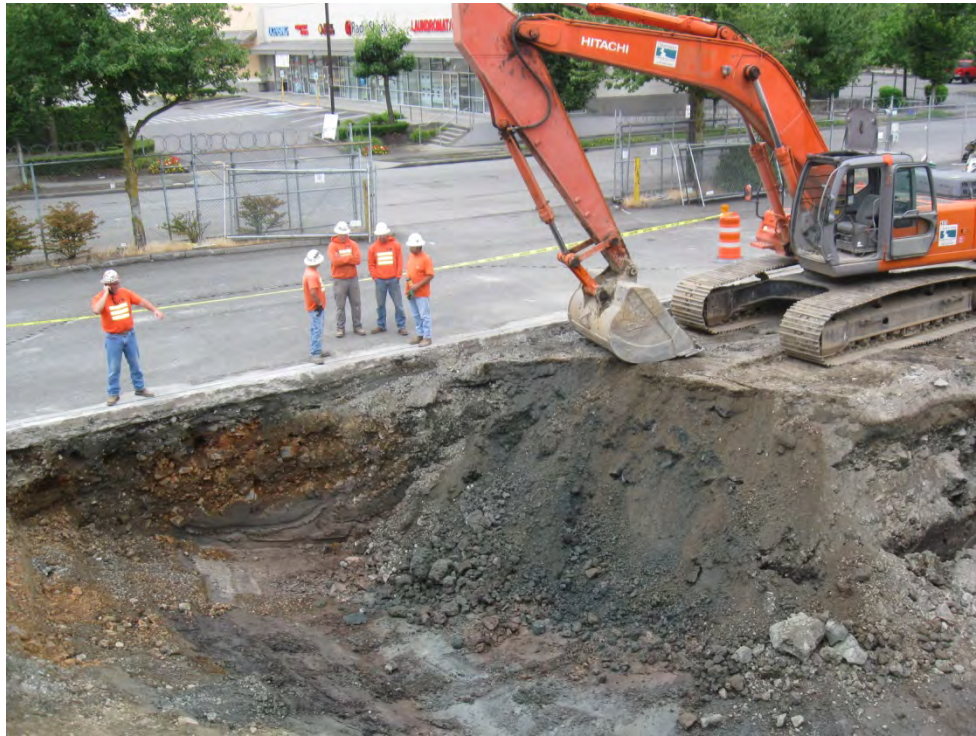
Photo 3: Excavation East of Former Monitoring Well MW02, 7/19/2011
