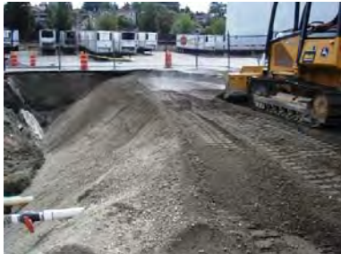
Type 17 Material Being Bladed And Water Being Added / East View
