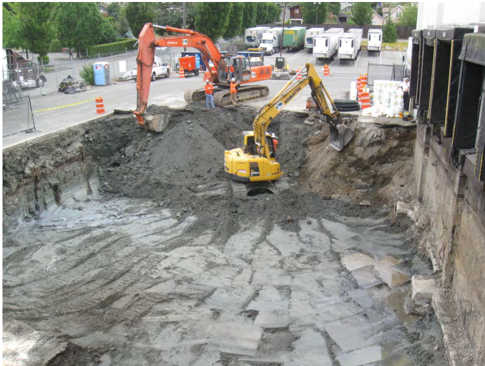
Photo 4: Excavation Showing Exposed North Wall Beneath Truck Bays, 7/20/2011
