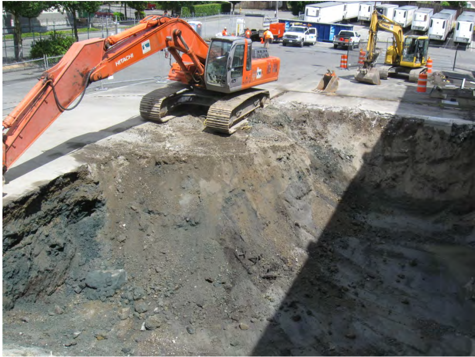
Photo 1: Initial Excavation in the Vicinity of Former Monitoring Well MW07, 7/16/2011
