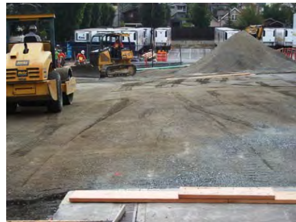
Type 17 Material Being Rolled and Compacted / East View
