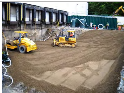
Starting back-fill operations at -11ft
