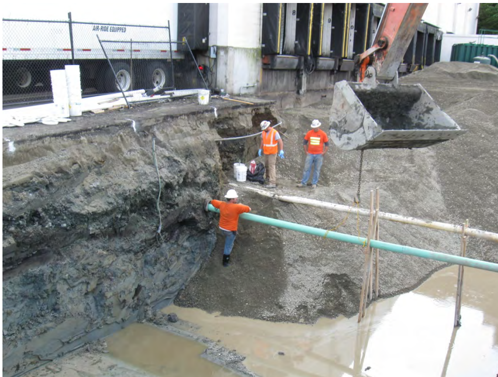
Photo 8: Storm Drain Line Replacement (Green Pipe), 7/26/2011
