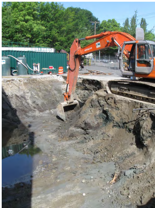
Photo 2: Southwest Corner of Excavation with Water Treatment System in Background, 7/18/2011
