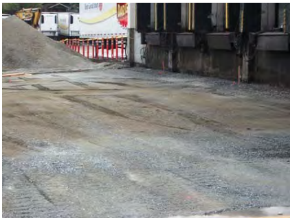
Type 17 Import Material At the North Loading Dock Area
