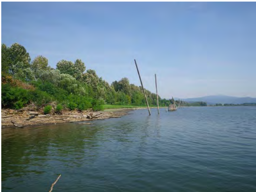
Photo 3. Southern edge of the project area along the Columbia River. The view is towards the east-northeast.
