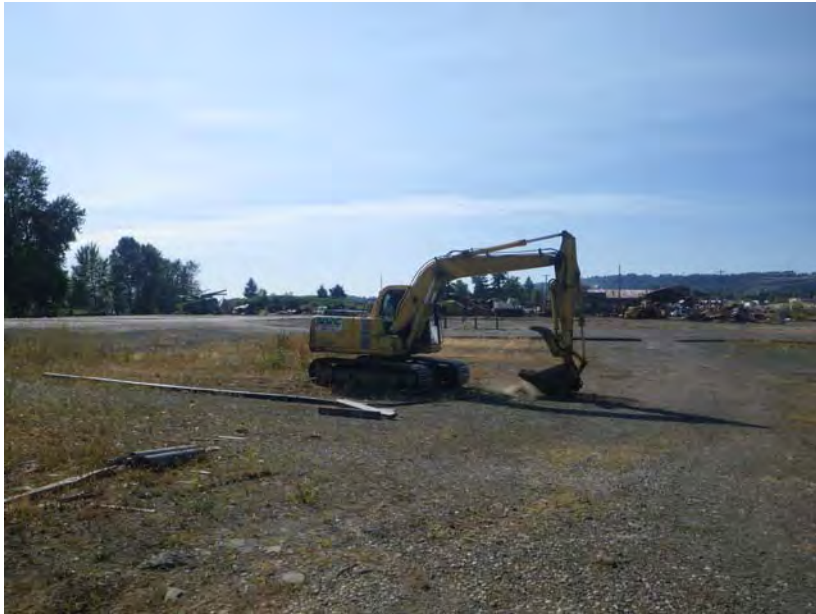
Photo 1. Excavation of test pit TP-8 within the Port of Camas-Washougal's Waterfront Brownfield Integrated Plan project area. The view is towards the southwest.
