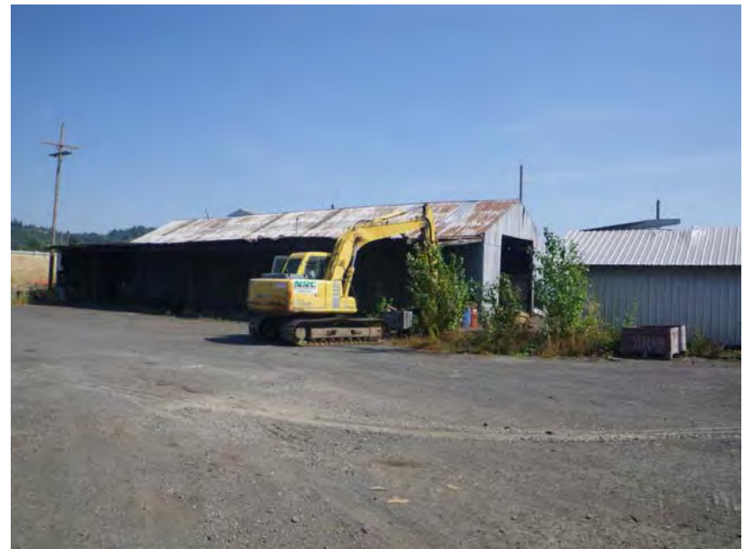
Photo 4. Corrugated metal building within project area. The view is towards the northeast.
