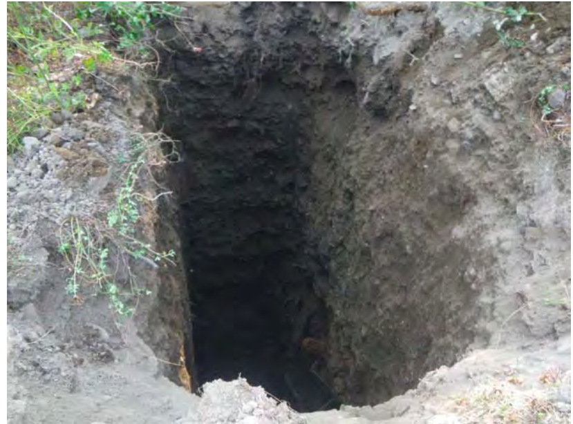
Photo 6. Test pit TP-6 at the end of excavation at a depth of 4.9 m (16.0 ft). The view is towards the north.
