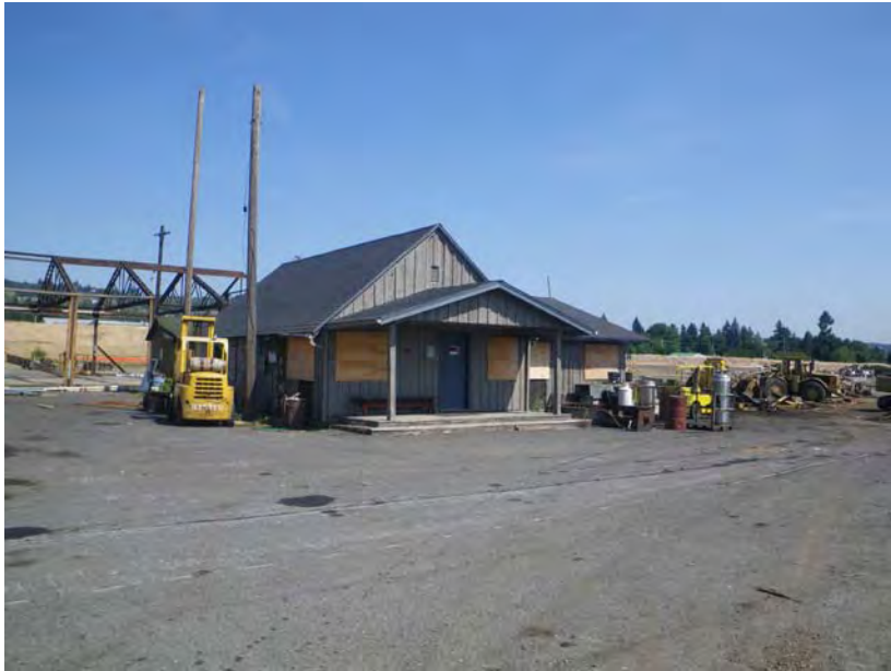
Photo 5. Shop or storage building within the project area. The view is towards the northeast.
