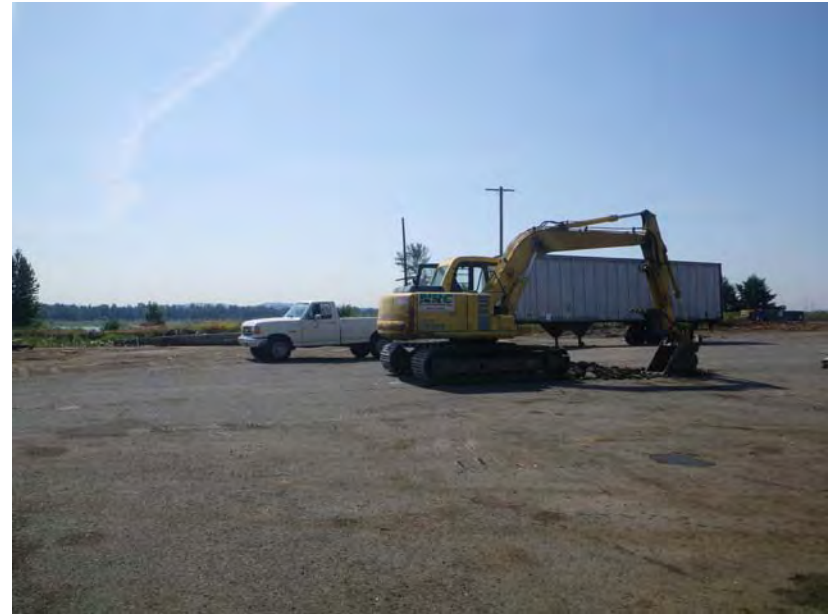
Photo 2. Excavation of test pit TP-10. The Columbia River is in the background to the left. The view is towards the south-southwest.
