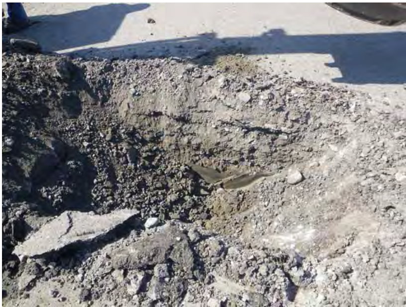
Photo 7. Excavation of surface soil sample SS# 20-1 at end of excavation at a depth of 0.9 m (3.0 ft). The view is towards the west.
