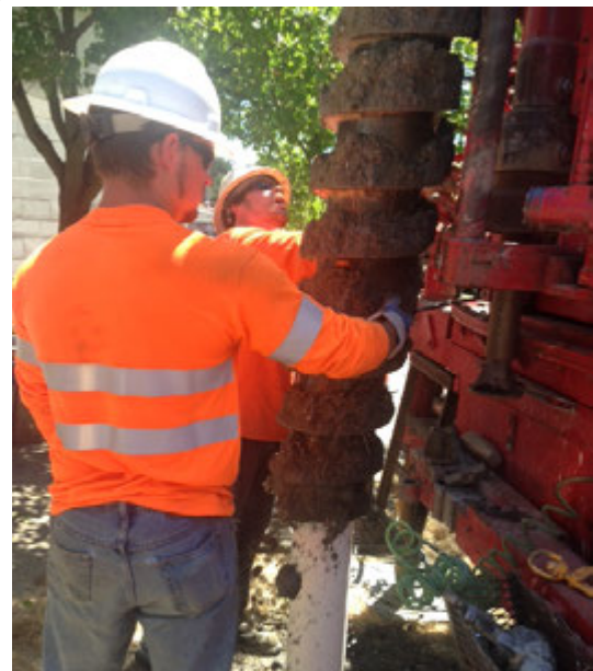
Installing MW-9R for petroleum contamination removal.
