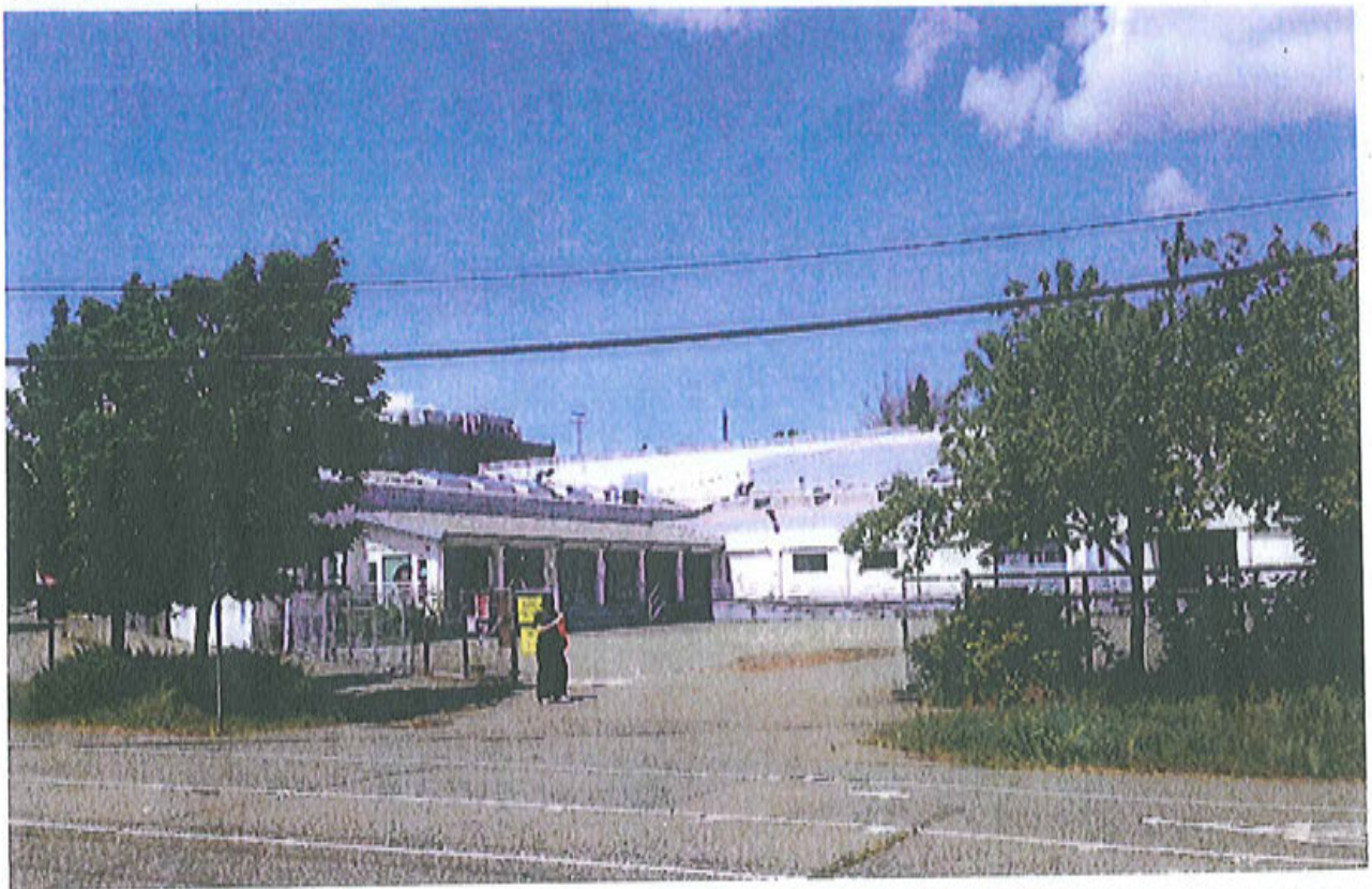
Figure 6. View looking north at Metro Transit Facilities North- North Yard and former Chevron Bulk Terminal #100-1327 with N Northlake Way and biking-pedestrian Burke-Gilman Trail in foreground with one pedestrian.
