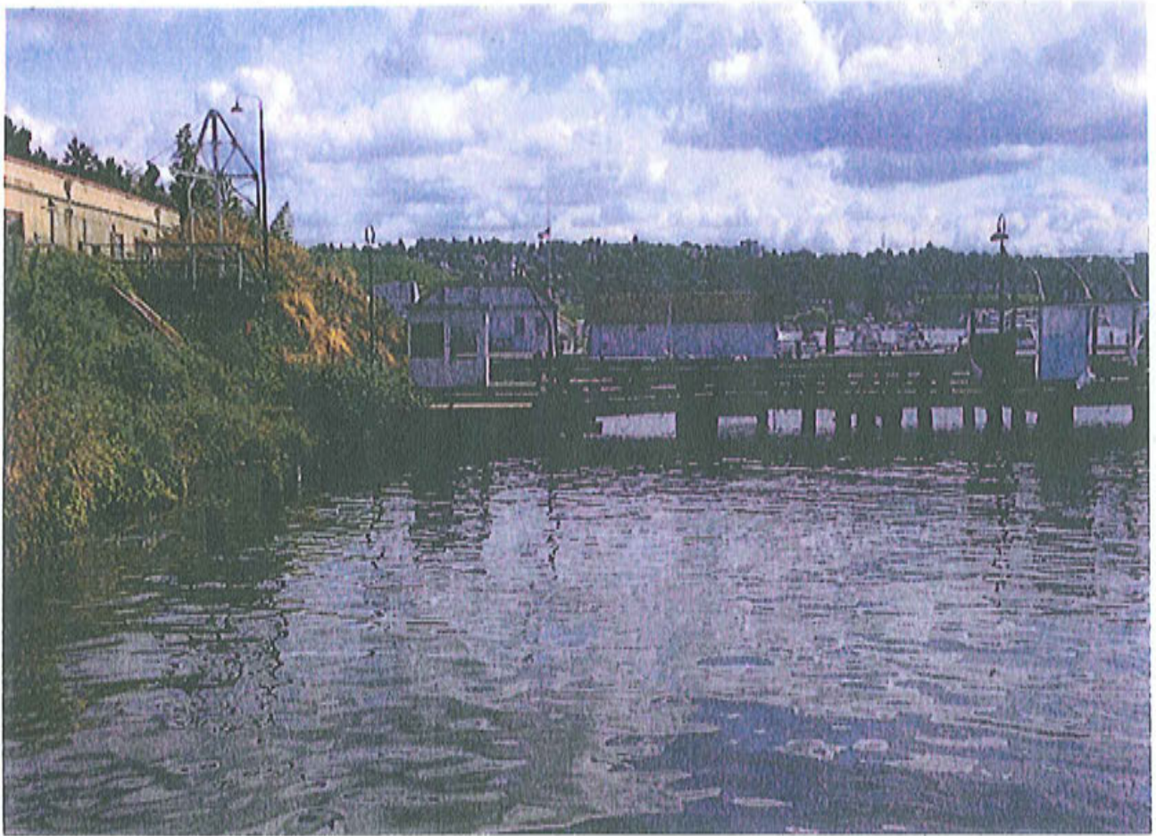
Figure 13. View looking east to former Metro Lake Union Site South Yard shoreline and one of two docks and warehouse in background to left.
