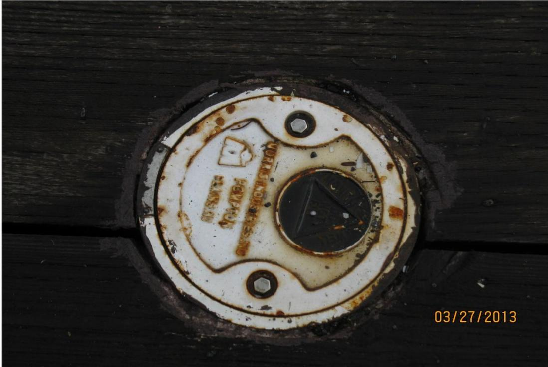
**Photo 6: Groundwater Monitoring Well AC-5**
