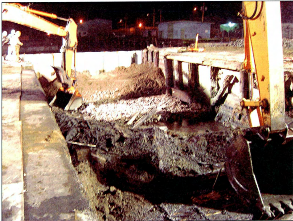
16. Marine railway well excavation/backfilling on January 20, 2004.
