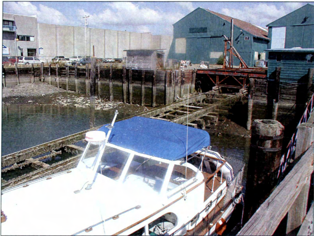
3. Old timber bulkhead and marine railway well.
