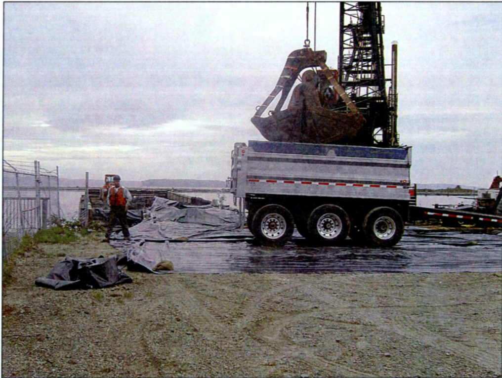
14. Sediment offloading at American Construction's south yard.
