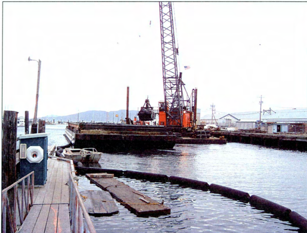
8. Sediment dredging and barge loading.
