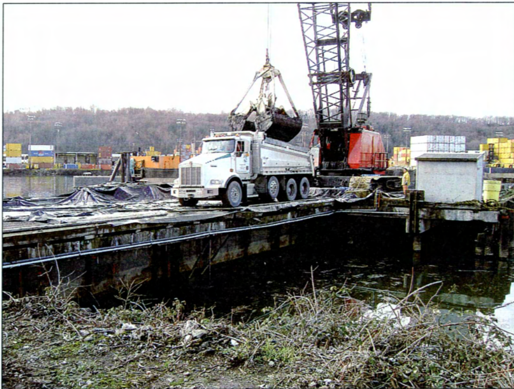
12. Sediment offloading at Alaska Logistics facility.
