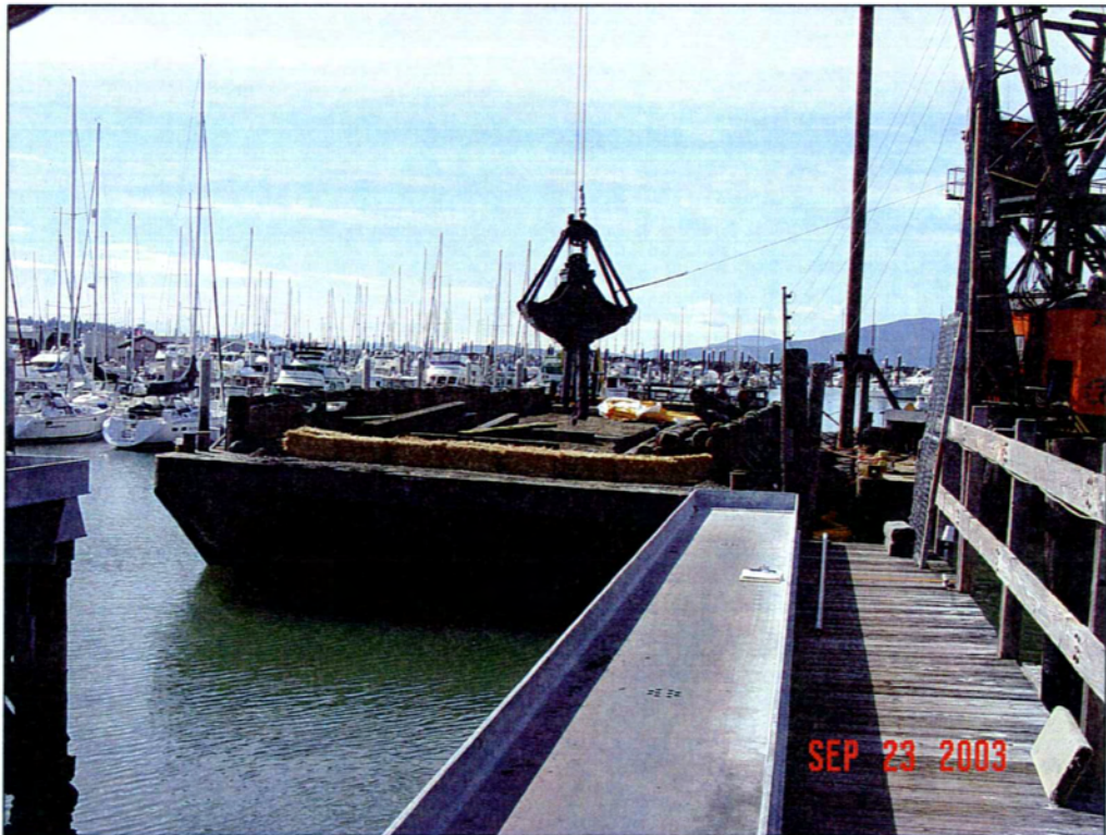
6. Marine railway demolition debris.
