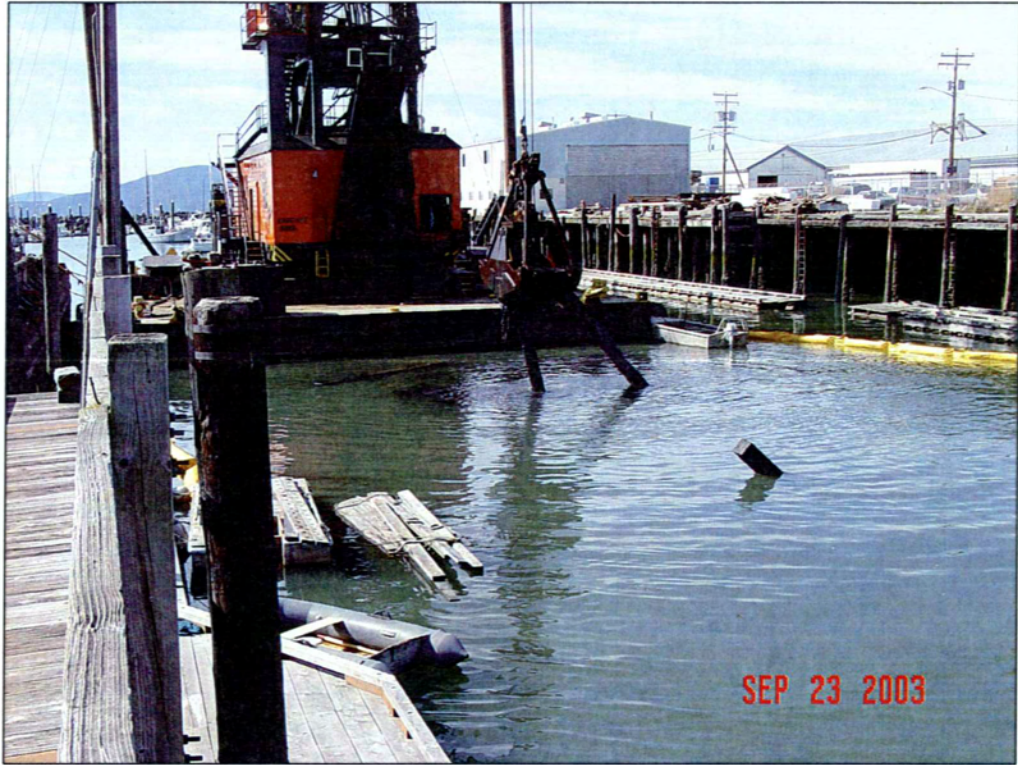
5. Marine railway demolition.
