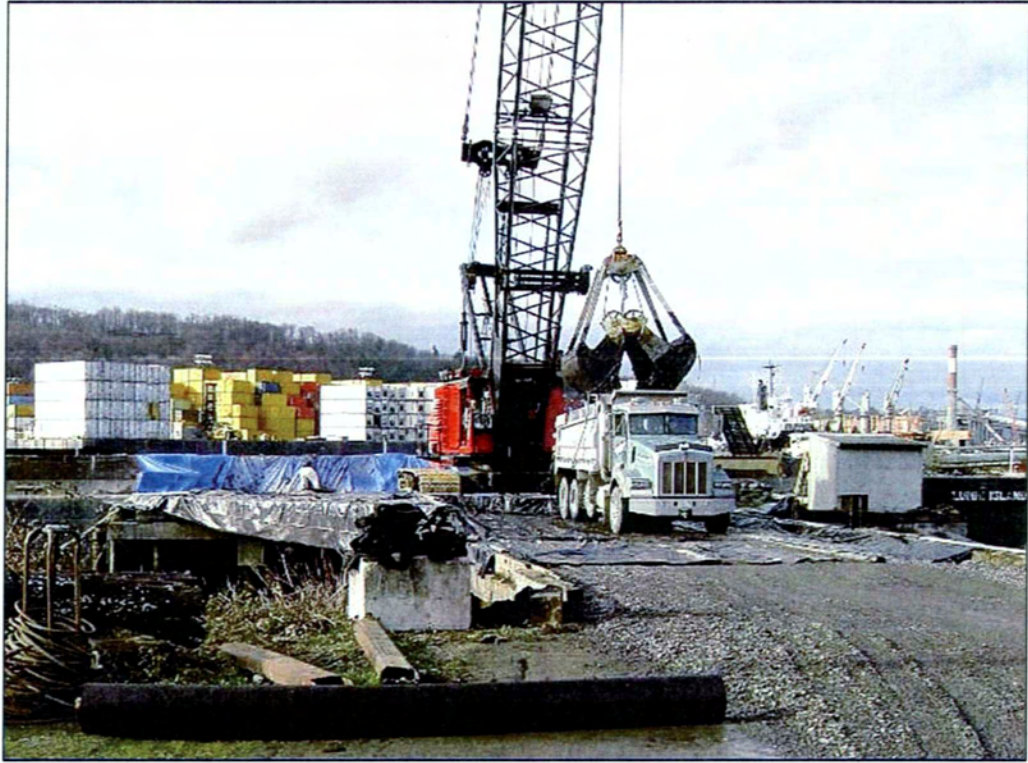
13. Sediment offloading at Alaska Logistics facility.
