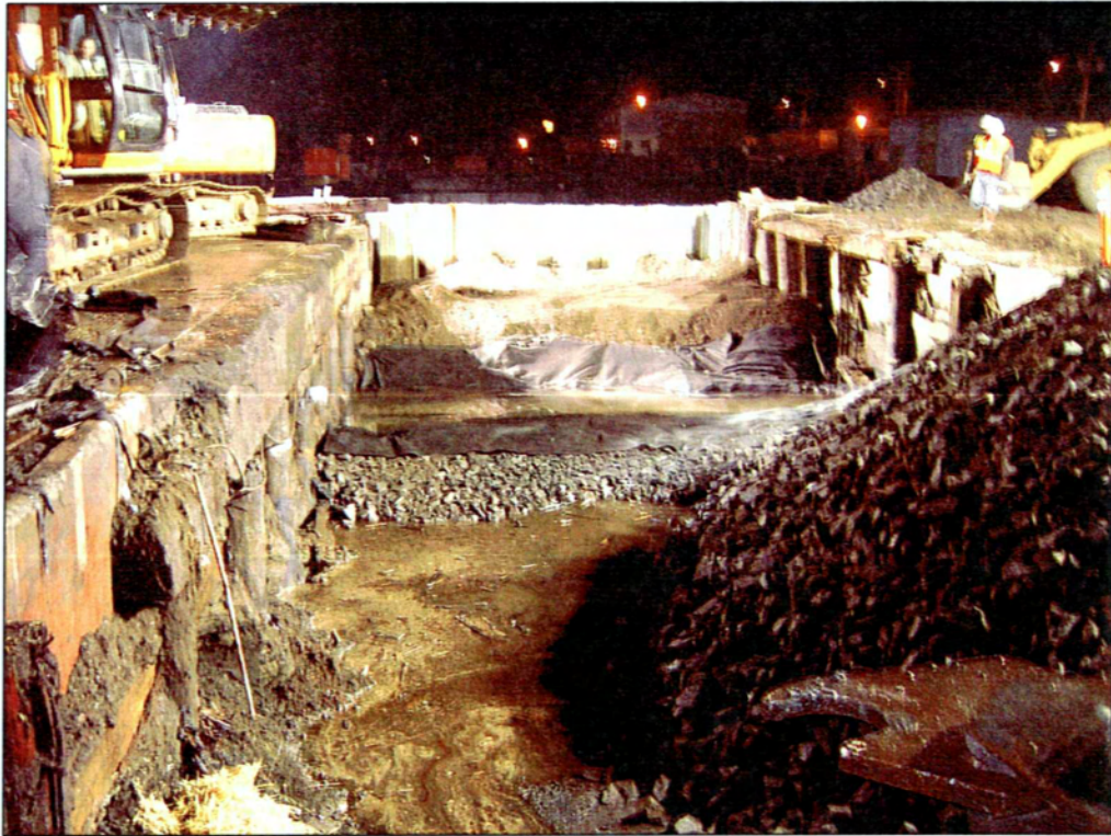
17. Marine railway well excavation/backfilling on January 21, 2004.
