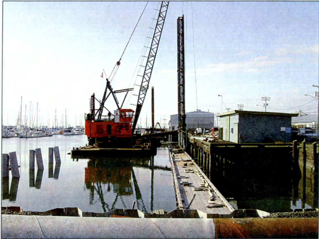
31. Installing new AZCA-treated fender piles along Segment C wharf.
