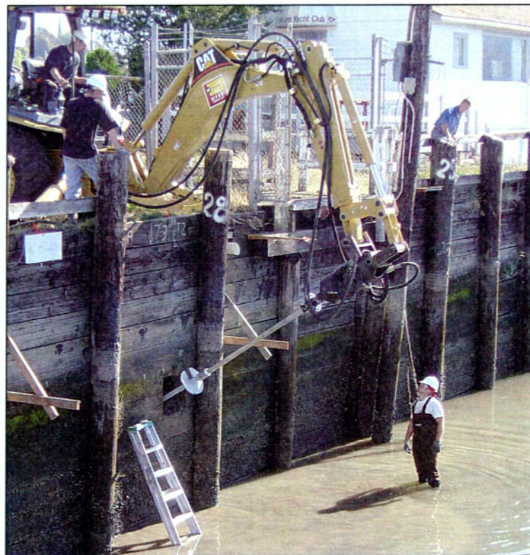
22. Helical tieback anchor installation for new bulkhead.
