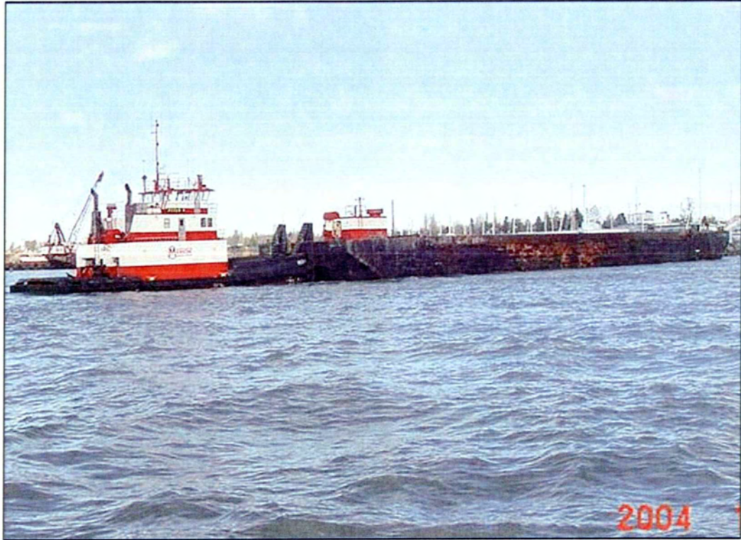
19. Marine habitat bench construction.
