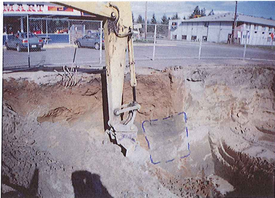
Photo 11 - View of north wall showing residual pocket of contamination from 6' to 13' BGS. Brown soil on top is "clean". Trail Mart is store behind excavation (02/28/96).
