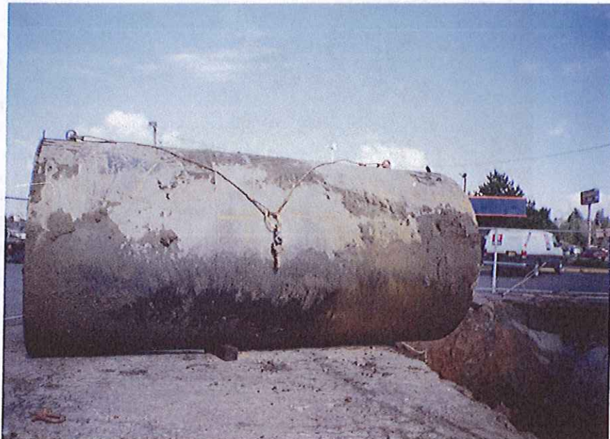
Photo 4 - View of tank T1 after excavation. The tank was found in good condition with no holes or pitting, and only minor rust (02/23/96).
