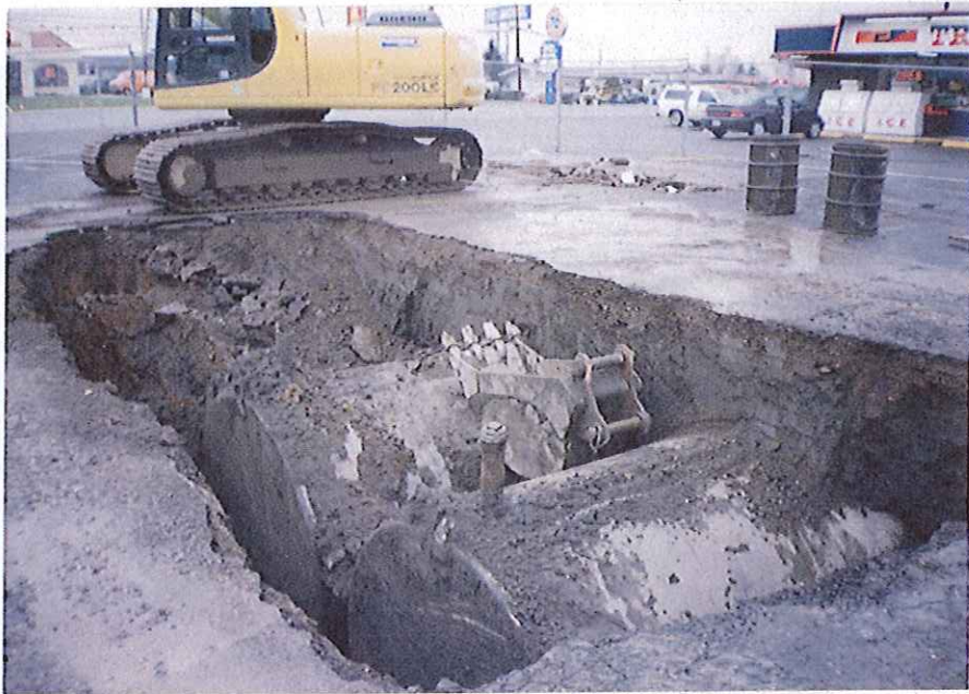
Photo 2 - West view of exposed tanks T1 (right), T2 (middle), T3 (buried on left) prior to excavation. Grey petroleum stained soil on right side of photo (02/21/96).
