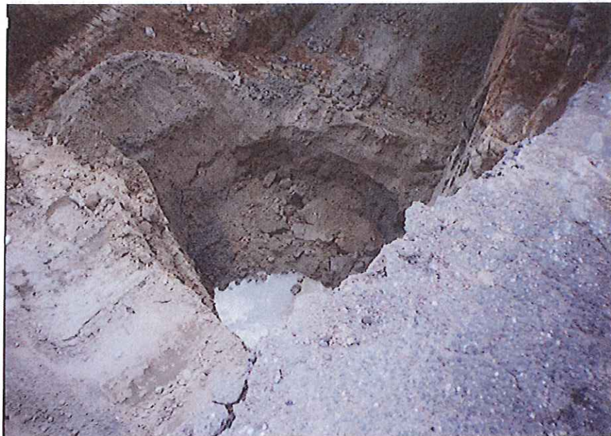
Photo 10 - Groundwater was encountered at 20' BGS in excavation. Note thin oily sheen on pit water surface. Brown soil in photo is clean (02/28/96).
