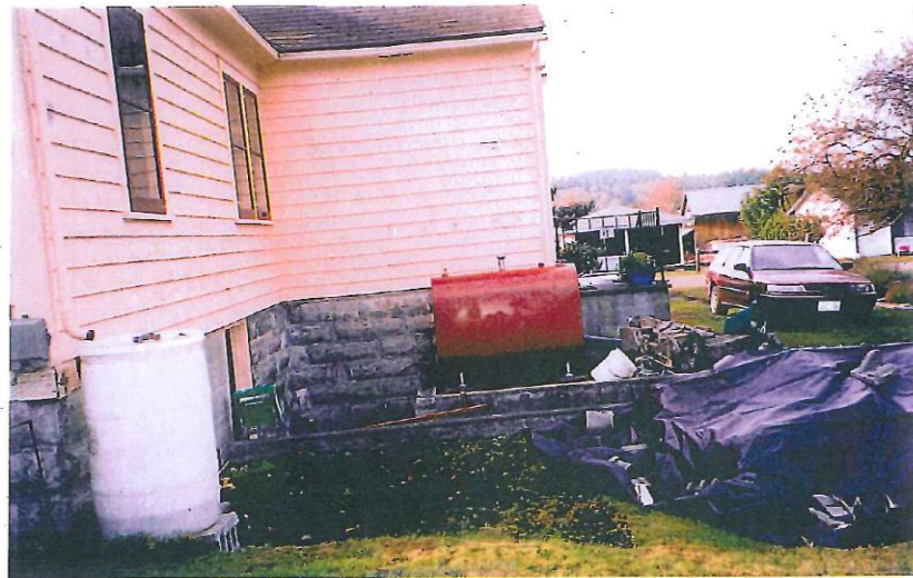
Photo 7: New Heating Oil Tank Installed
