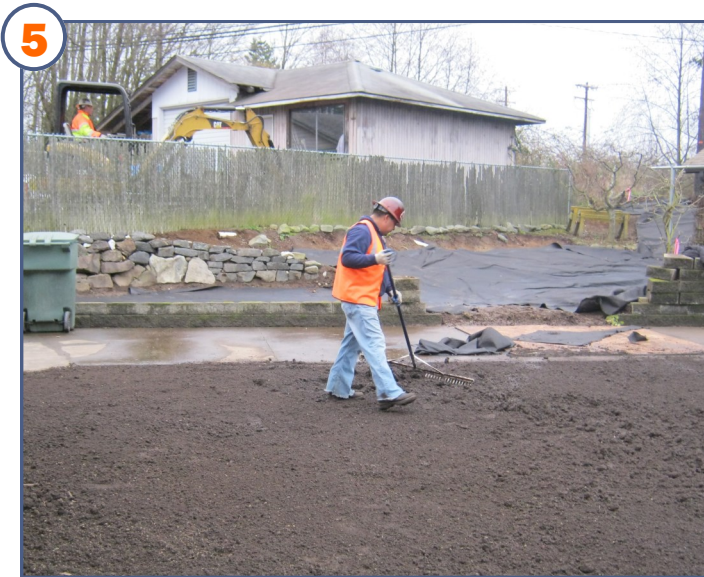
5 They spread the soil and level it to the pre-existing grade.
