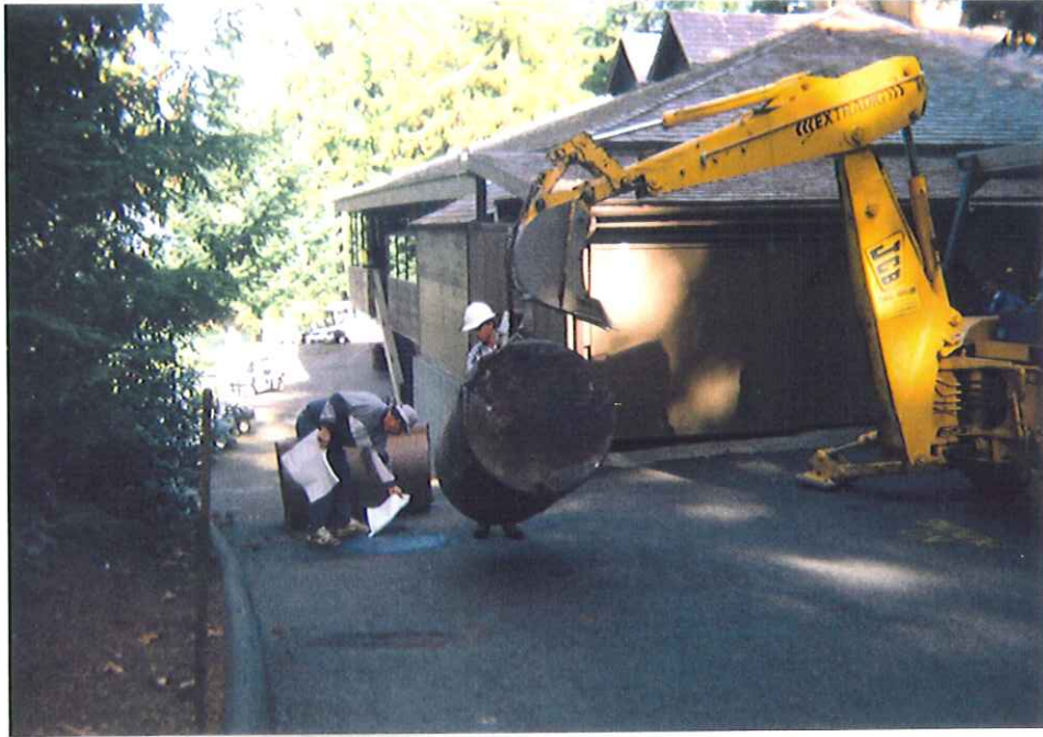
VIEW OF EXCAVATED TANK NEAR RESTAURNT/CLUB HOUSE
