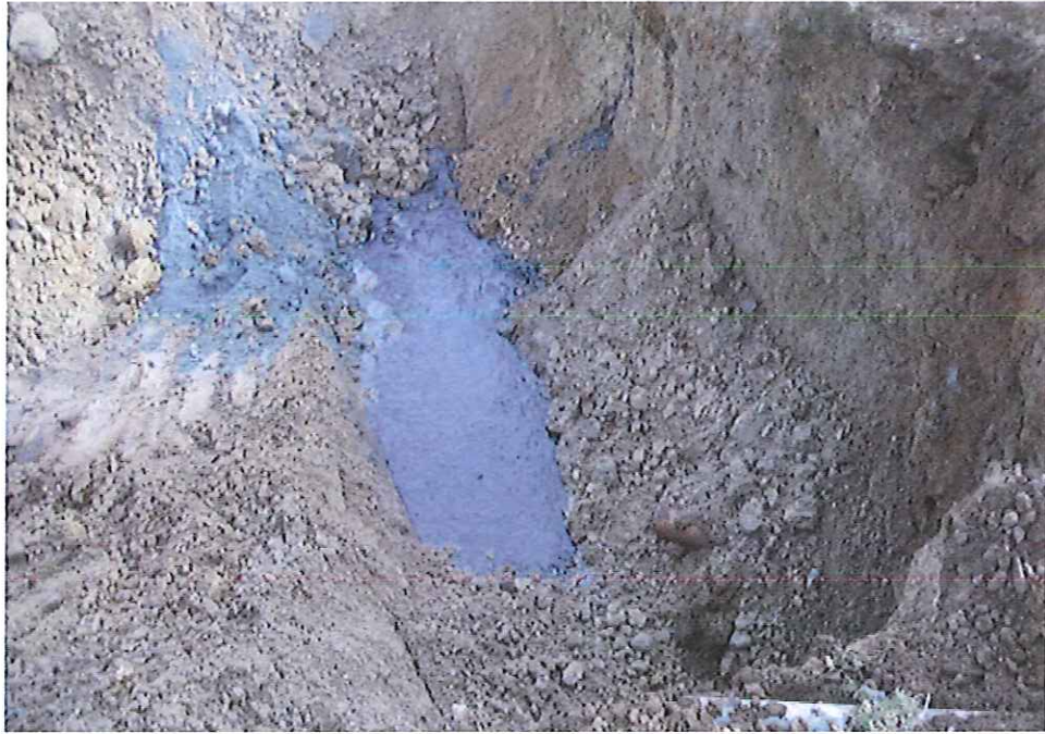
Looking west at the Holly building tank pit following removal. Obvious PCS noted.
