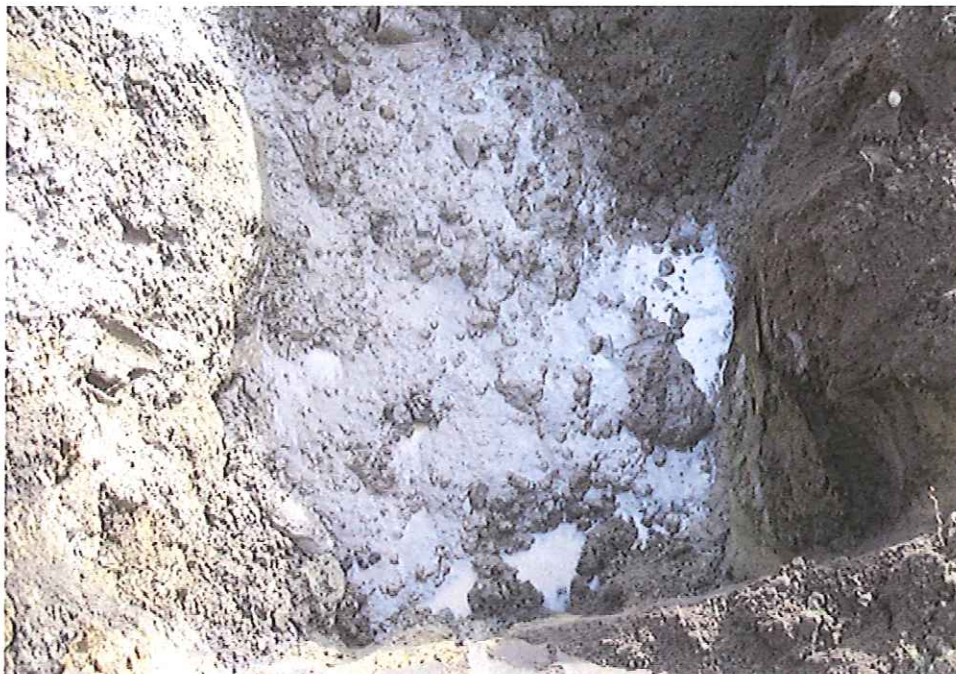
Heather building tank pit following removal. No visual or olfactory indications of PCS noted.
