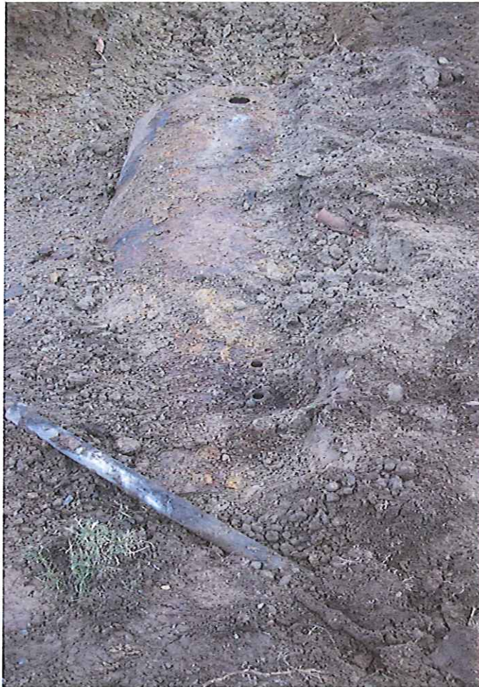
Holly building tank top exposed under 20" of asphalt and earth cover.
