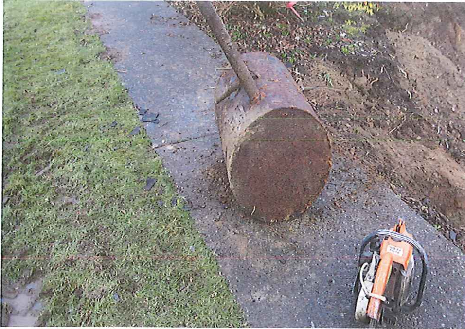
The removed starter tank was sized at 20" x 30", with a nominal capacity of 41 gallons.
