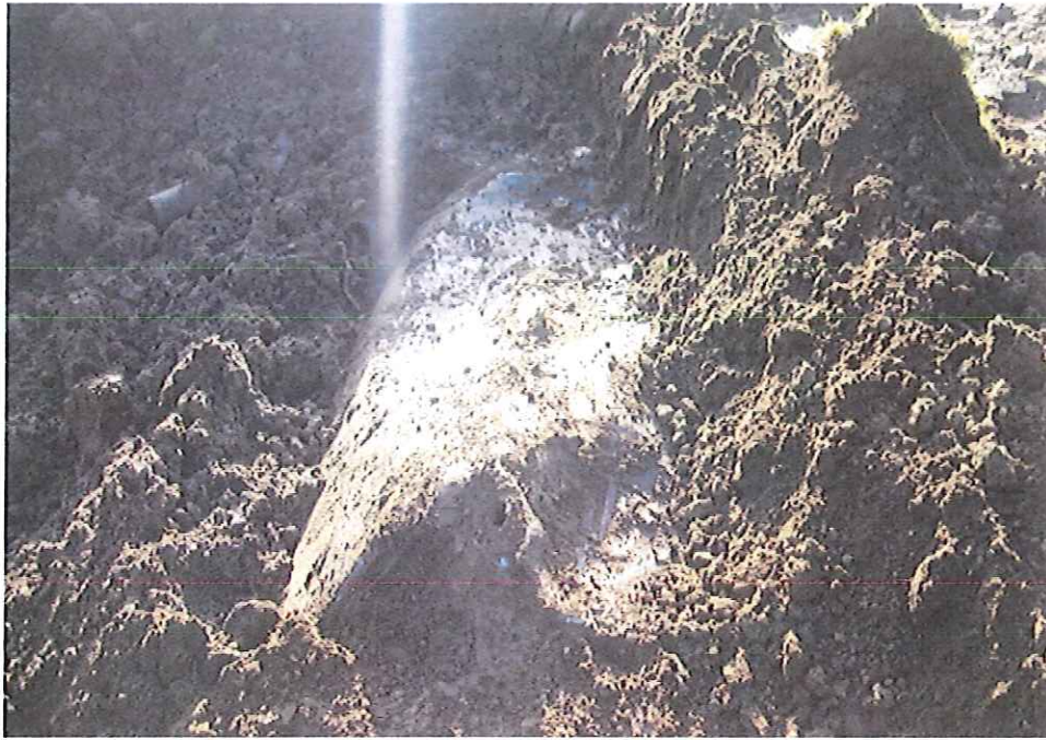
Gym tank top exposed under 30" of earth cover.
